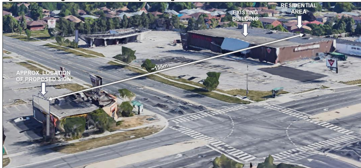
Figure 7: Existing barrier between Proposed Sign and residential area 155m to the northeast
