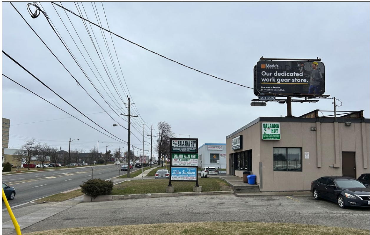
Figure 2: The Existing Two Sign Structures Currently in Place at the Subject Premises
