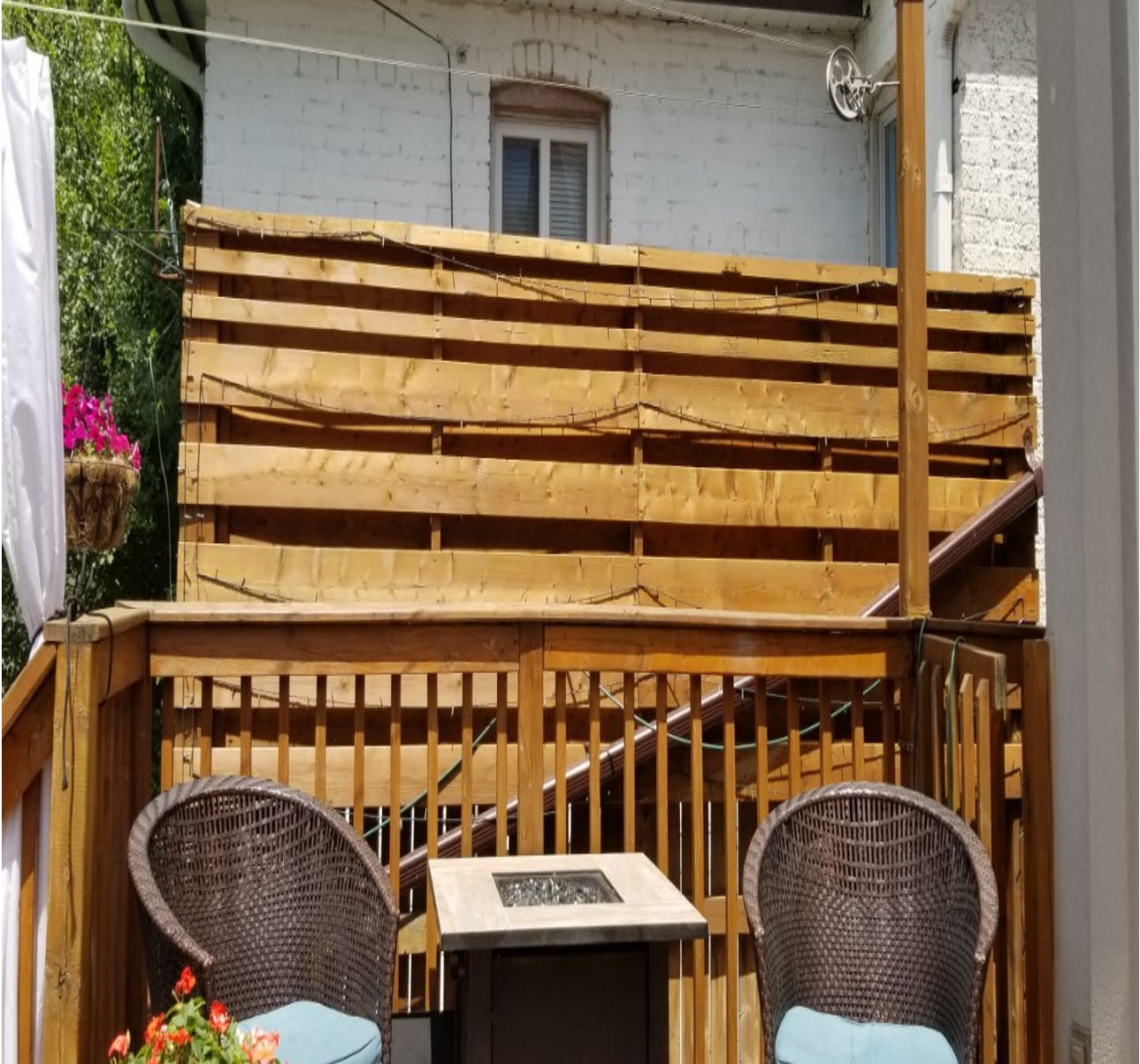
Attachment 3: Municipal Standards Officer's Photo 28 Byng Avenue – Rear Yard- North Side Fence
