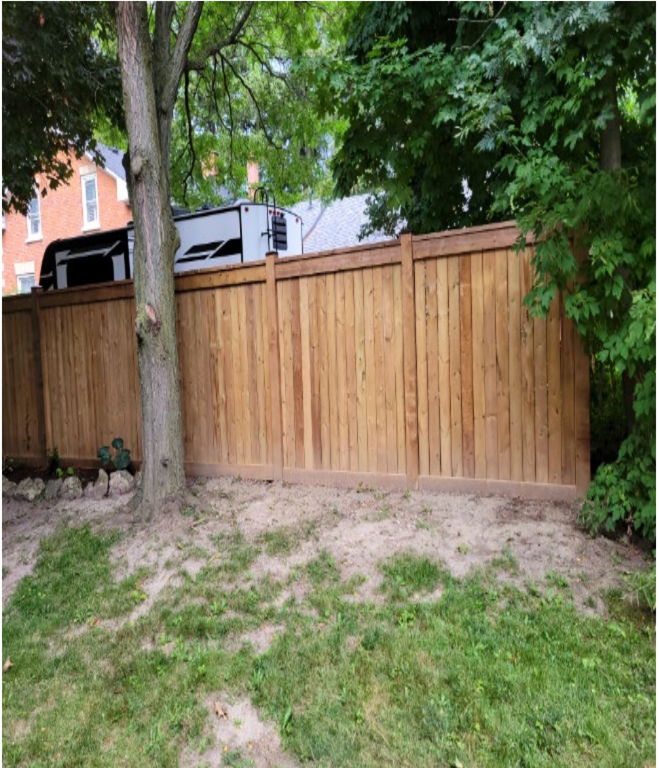
Attachment 2: Municipal Standards Officer's Photo - 20 Farmington Crescent - Rear Yard
