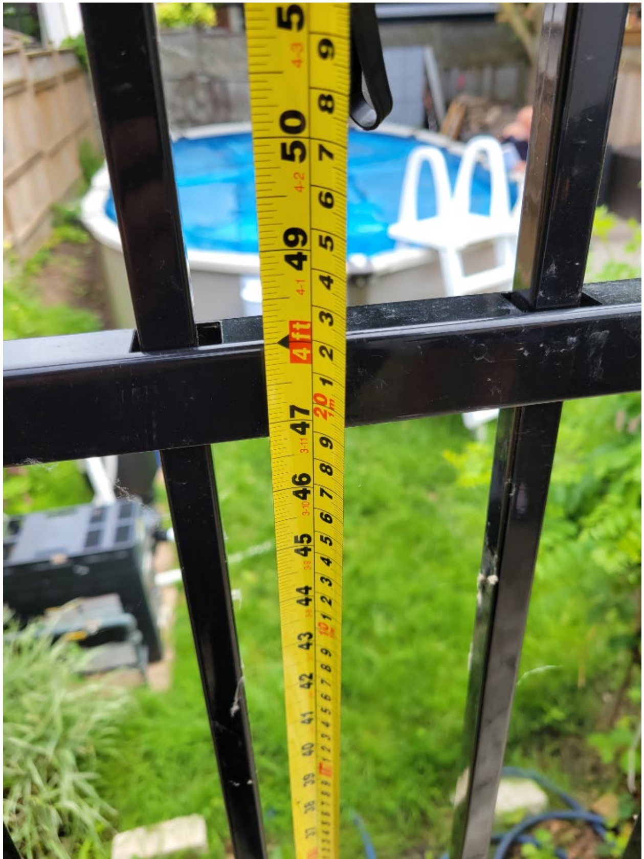
Attachment 6: Deck Guard Measurement
