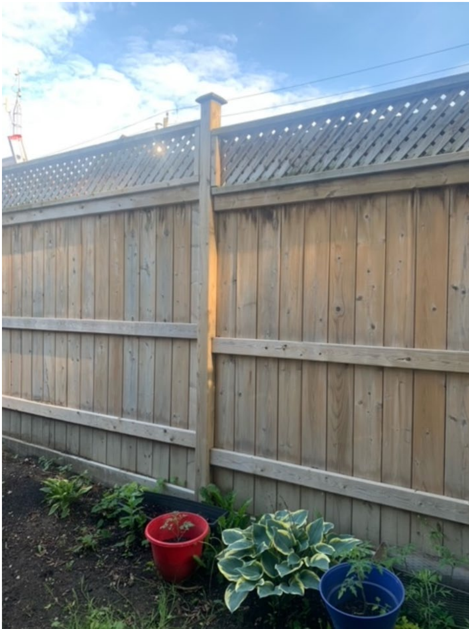
Attachment 2: Applicant Photo - rear yard north side fence
