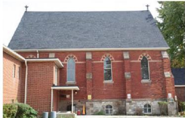
West elevation (source: HIA)
