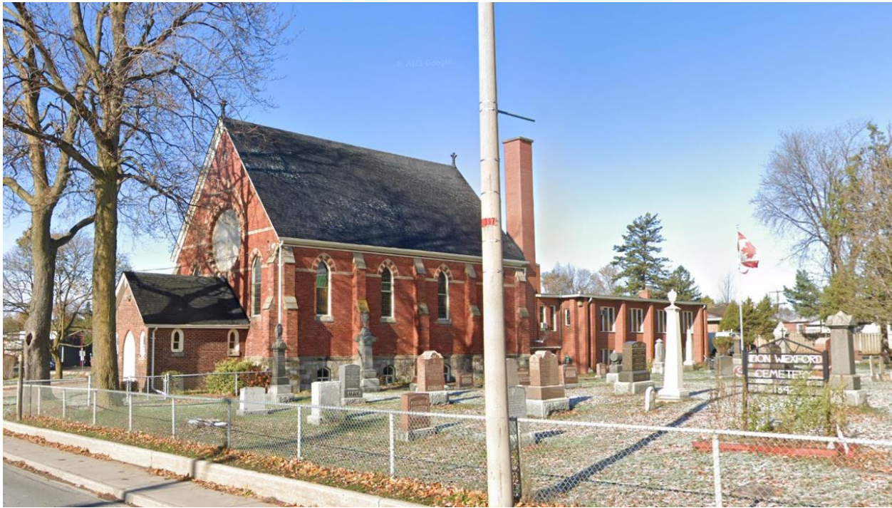
East elevation of historic church, addition at rear and cemetery (source: Google Maps)
