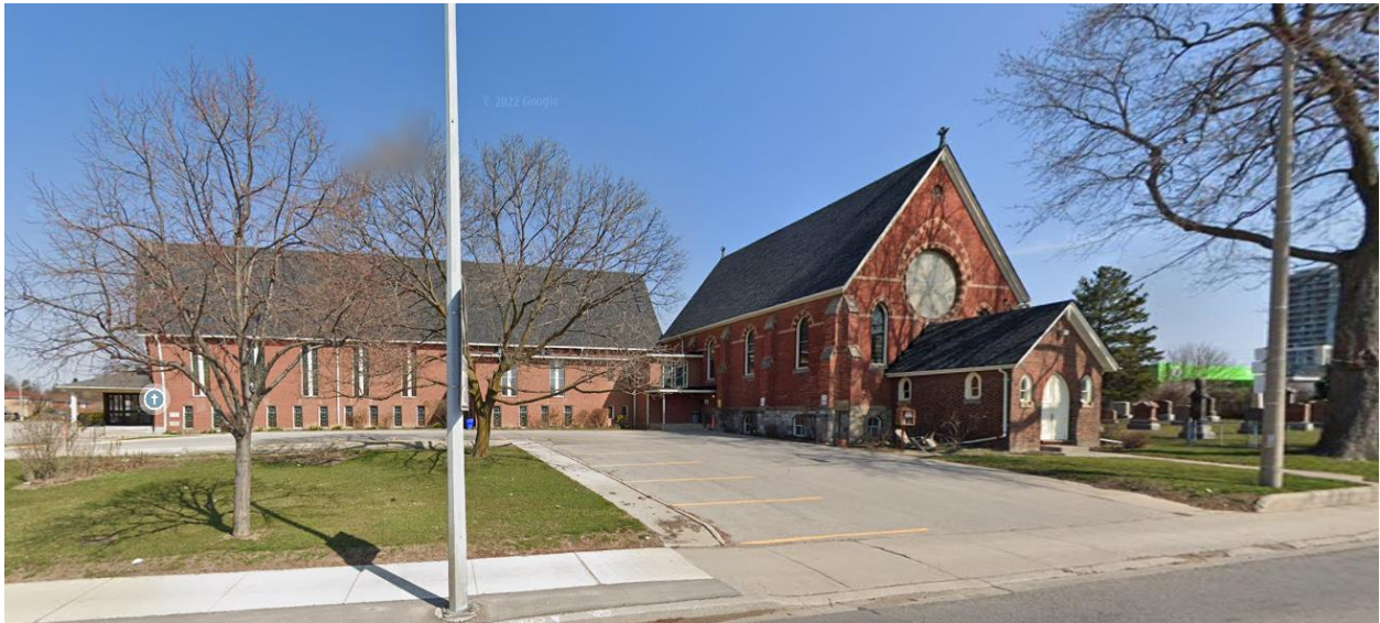
South and west elevations of historic church (right) and post-war addition (left) (source: Google Maps)
