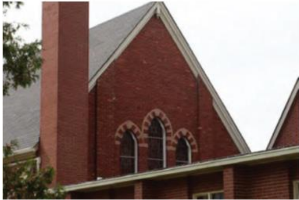
North elevation (behind addition) (source: HIA)
