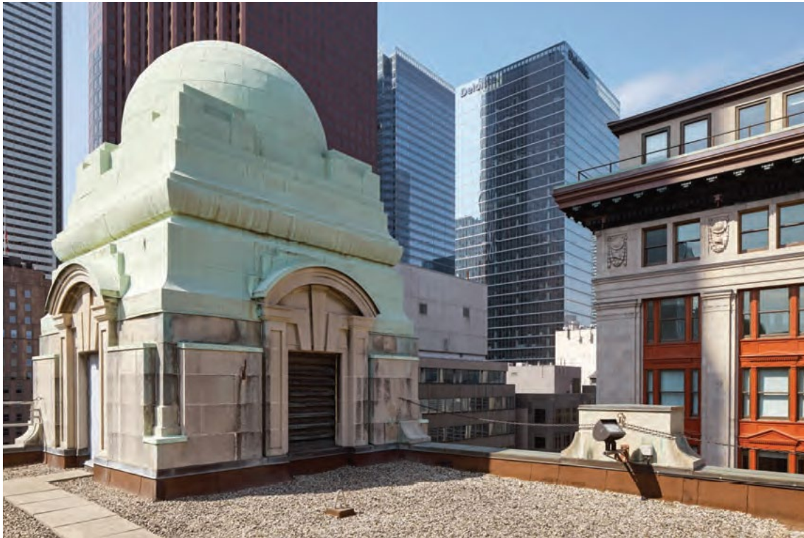
View of the north-west cupola (source: ERA HIA)
