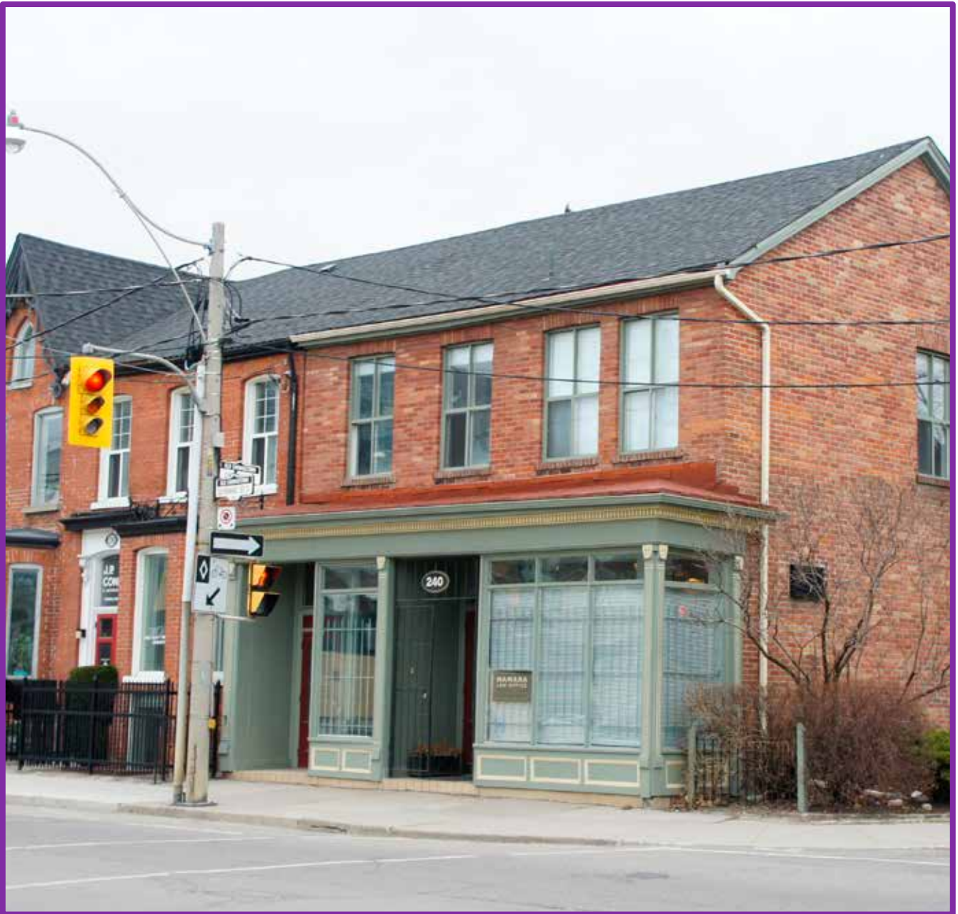
Figure 70: Historic storefront at 240 Gerrard St. E.
