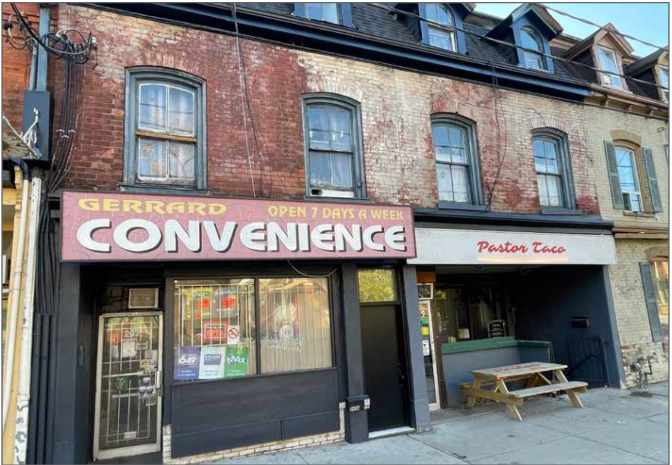
Figure 72: Gerrard St. E. storefront with non-historic finishes.
