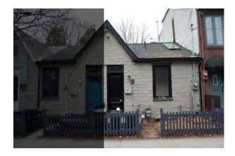
Materials Insulstone exterior cladding and asphalt shingle roofing
