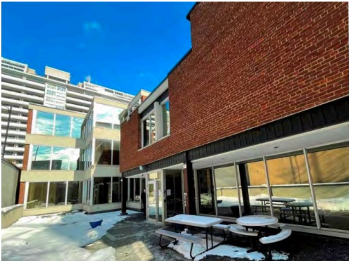
View of the west elevation with entrance, terrace and three-storey rear wing (Heritage Planning).
