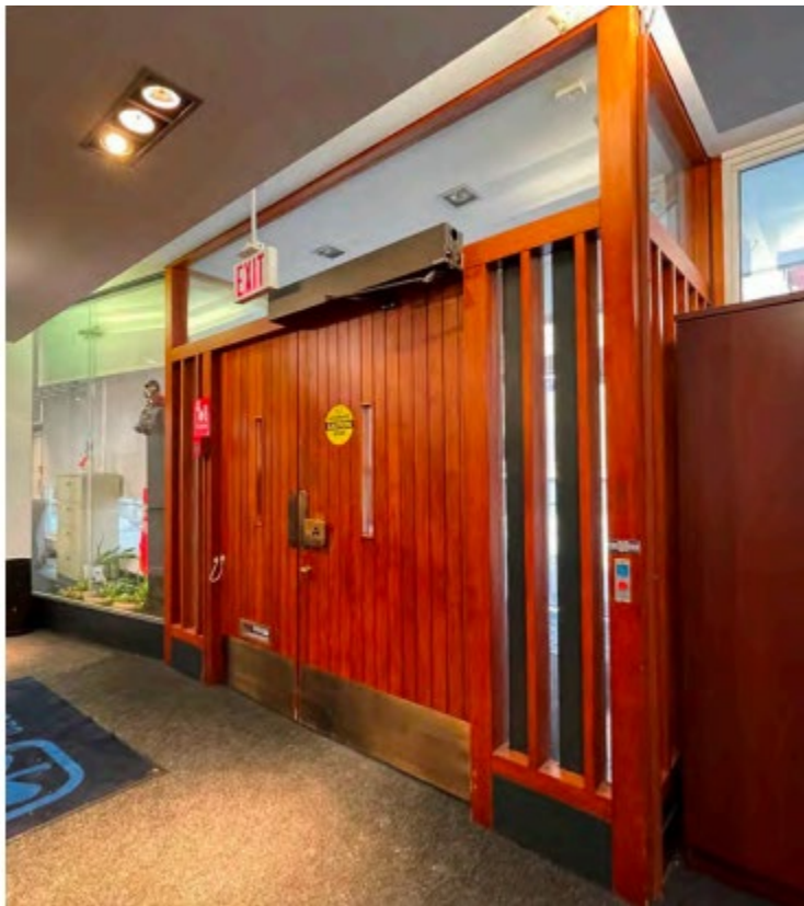
View of the wood-paneled doors with ironmongery door pulls (Heritage Planning).
