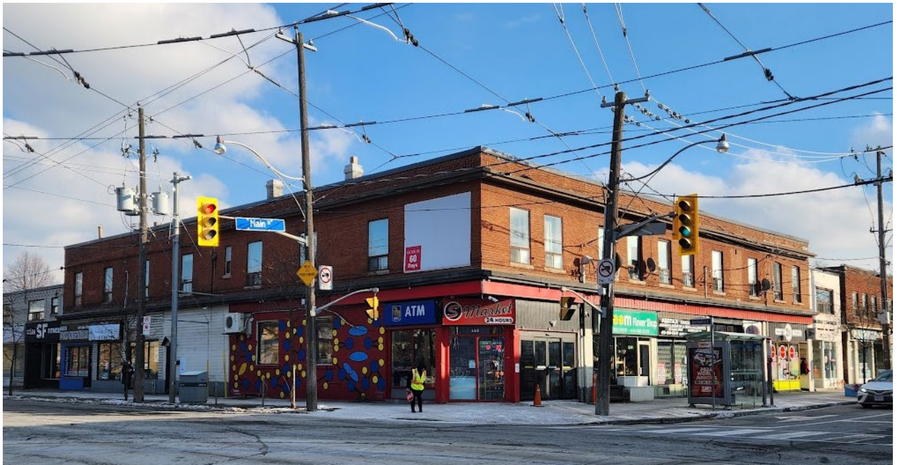
155, 161, and 167 Main Street and 2201, 2203, 2205, and 2207 Gerrard Street East, viewed from the northwest. Heritage Planning, 2024
