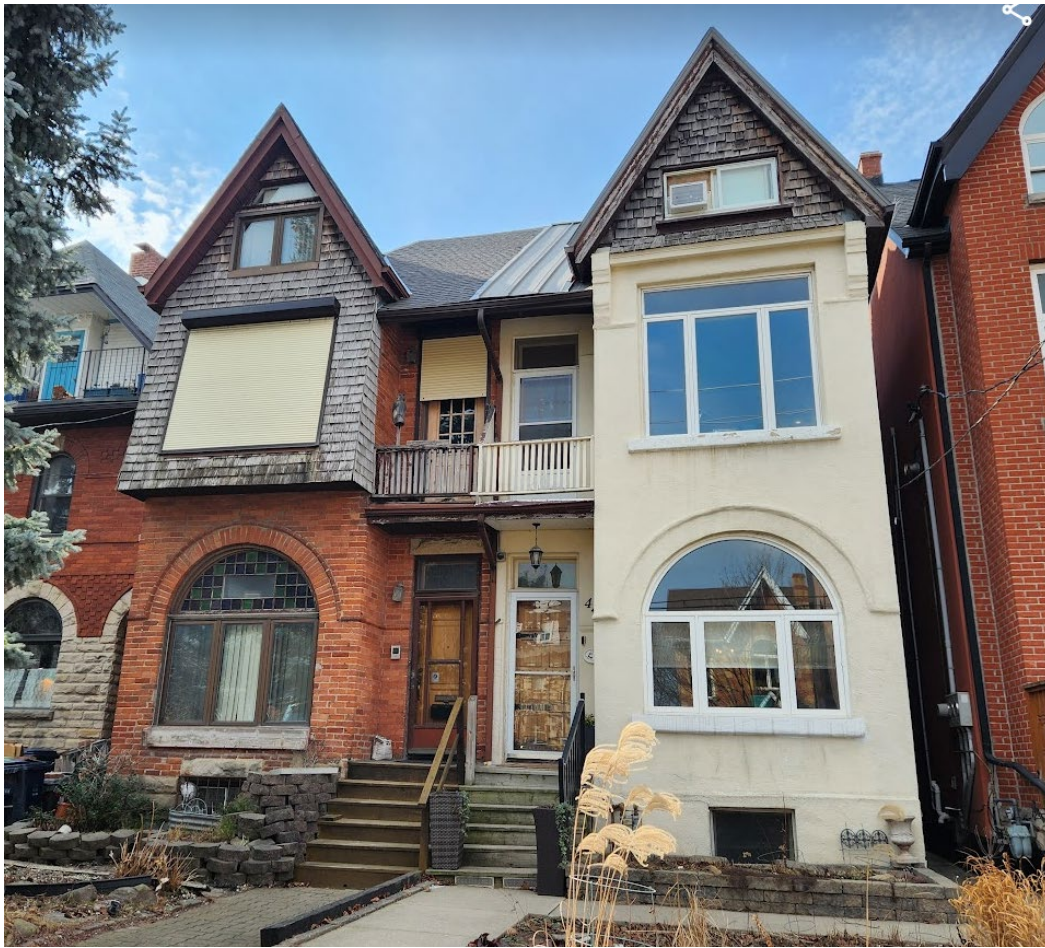
42 and 44 River Street, Heritage Planning, 2024
