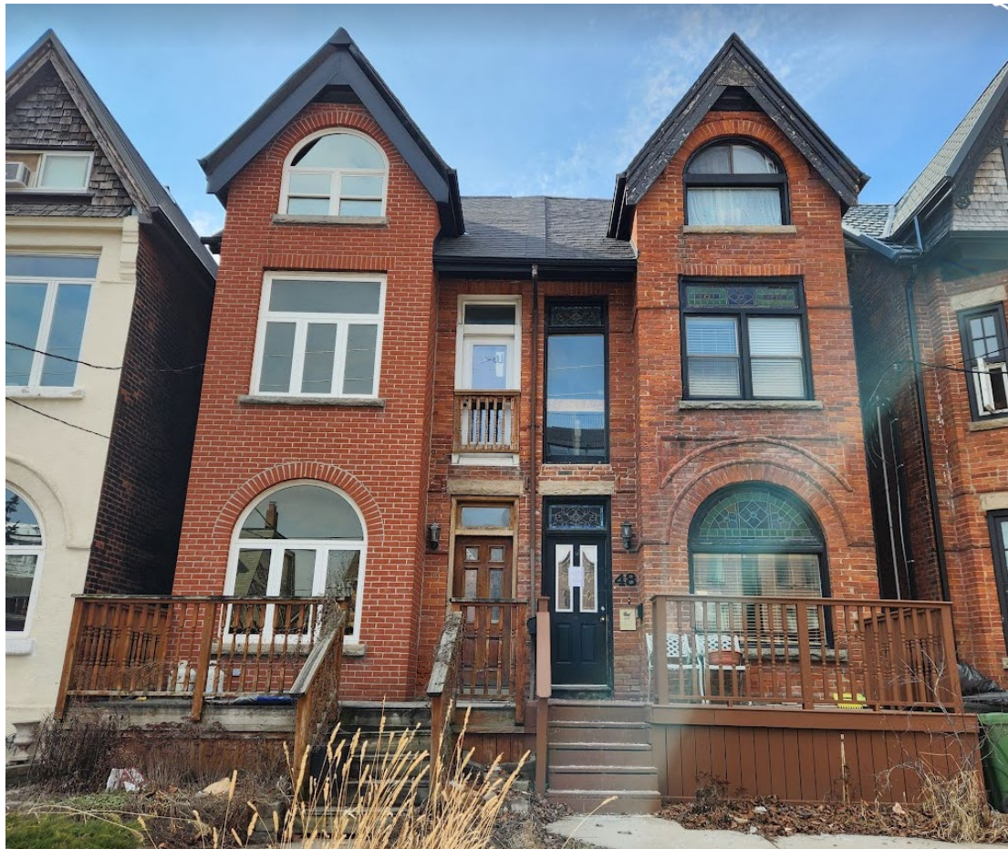
46 and 48 River Street, Heritage Planning, 2024
