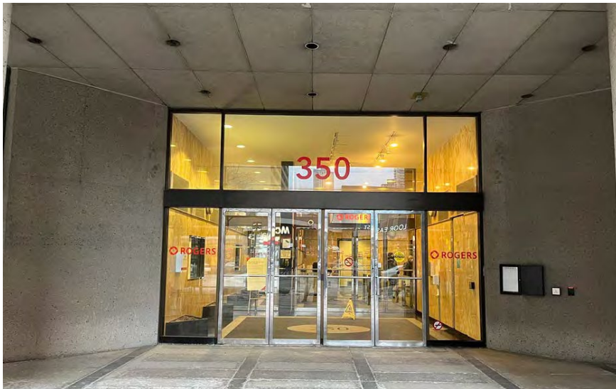
View of the primary entry of 350 Bloor Street East facing south.
