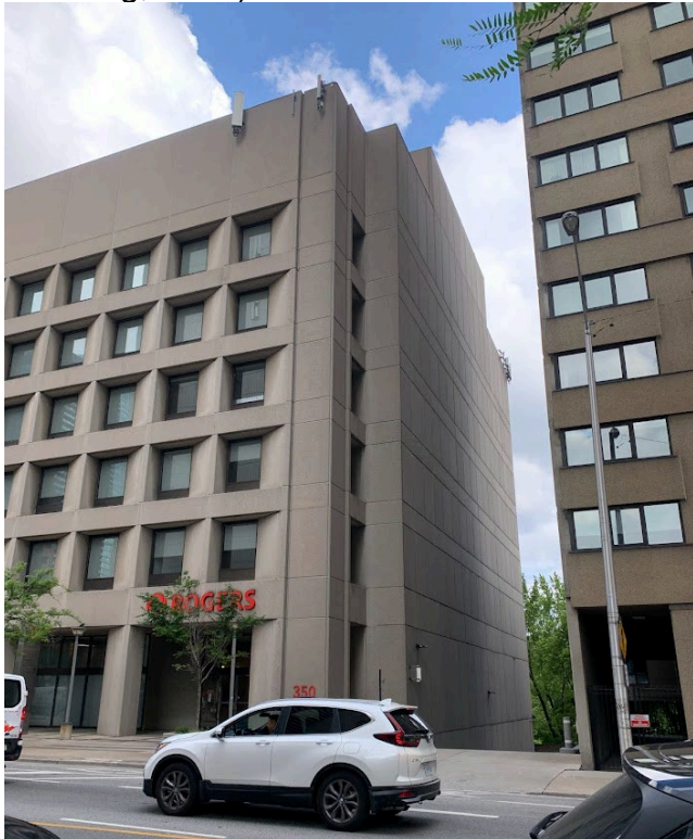
View of southwest corner of the building showing the east elevation with a predominant blank wall
