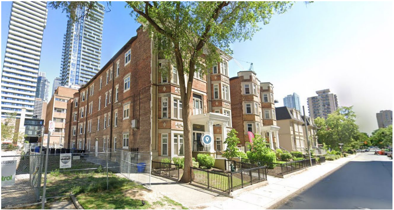
Contextual view of the southwest elevation at 36 Maitland Street (Google Maps, 2021).
