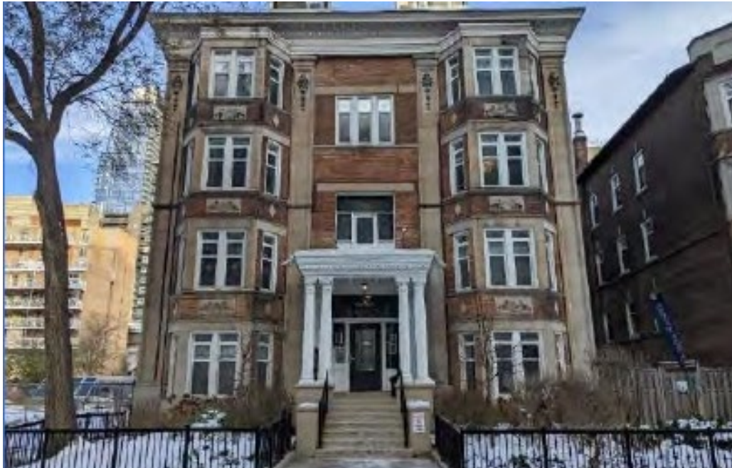
Contextual view of the south (primary) elevation at 36 Maitland Street (LHC Heritage Planning & Archaeology Inc, 2023).
