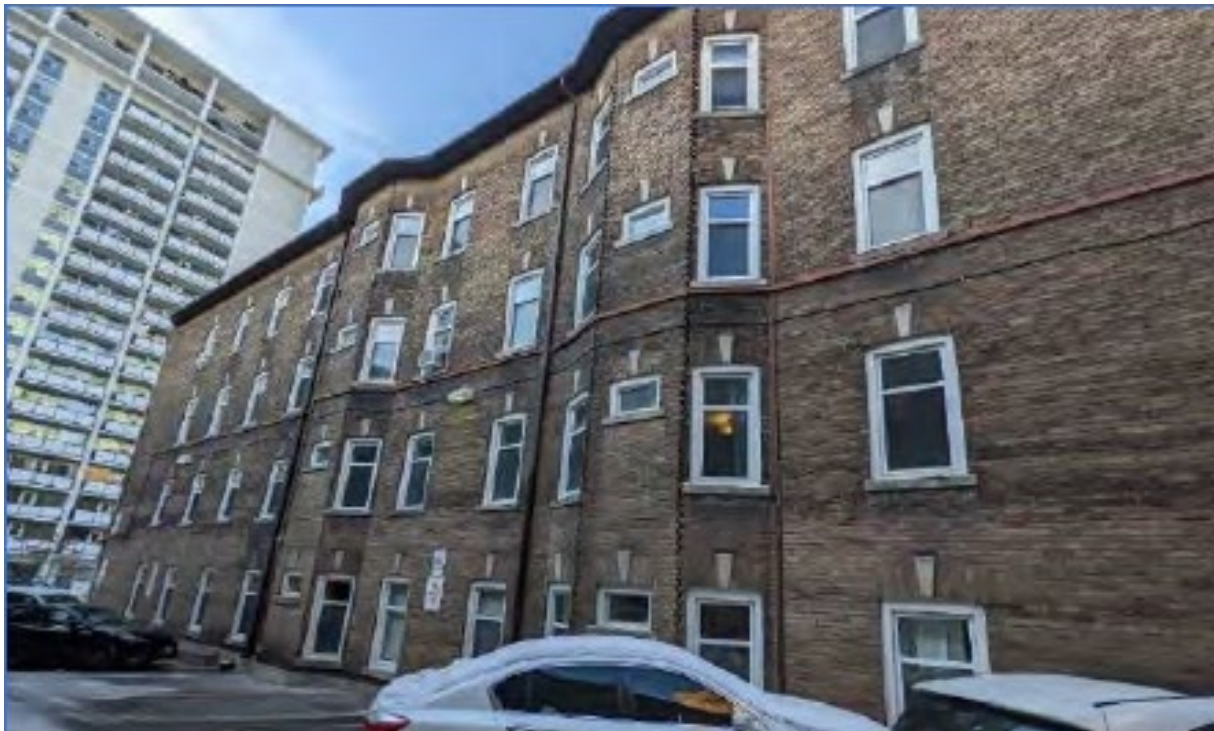
View of the east elevation at 42 Maitland Street (LHC Heritage Planning & Archaeology Inc, 2023).
