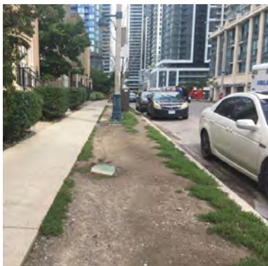
Photo of East Liberty Street boulevard needing repair due to worn-out sod and pedestrian volumes.
