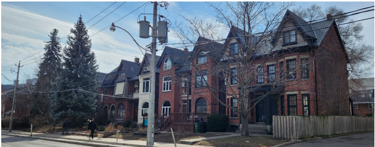
Streetscape formed by 34 to 52 River Steet, Heritage Planning, 2024
