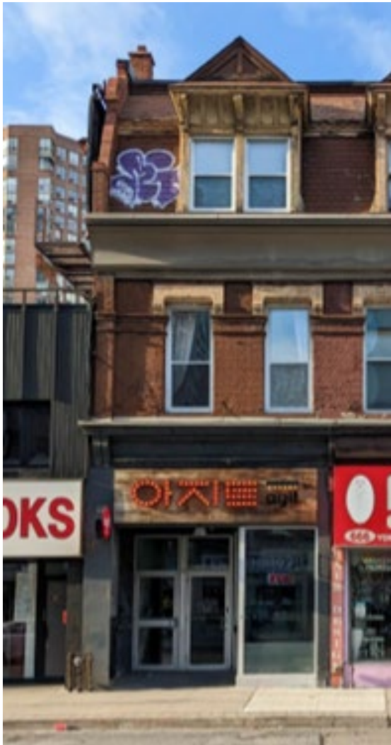
View of the east (primary) elevation of 664 Yonge Street (Heritage Planning)
