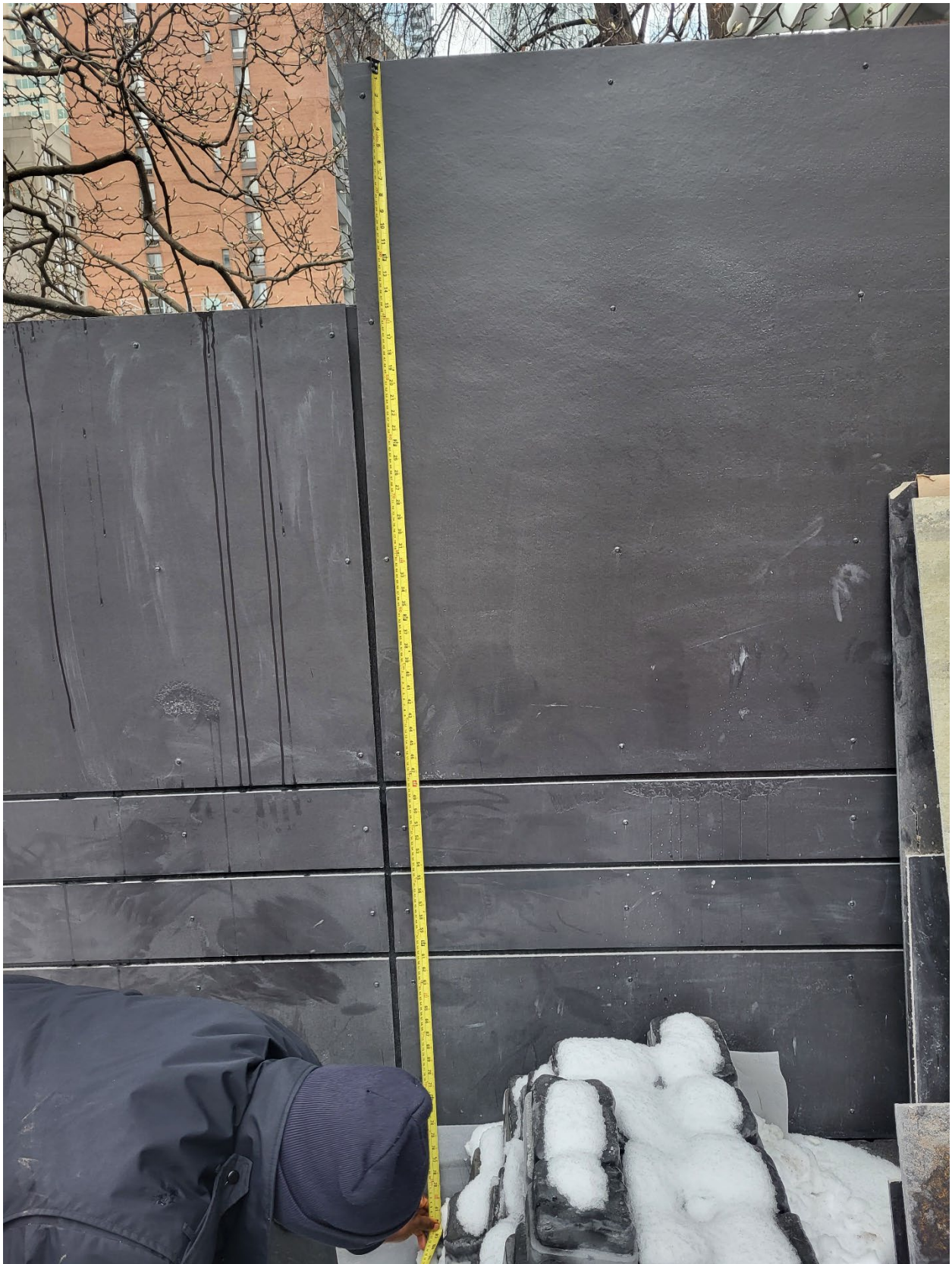
Attachment #2: Measuring of fence located on 137 Collier Street
