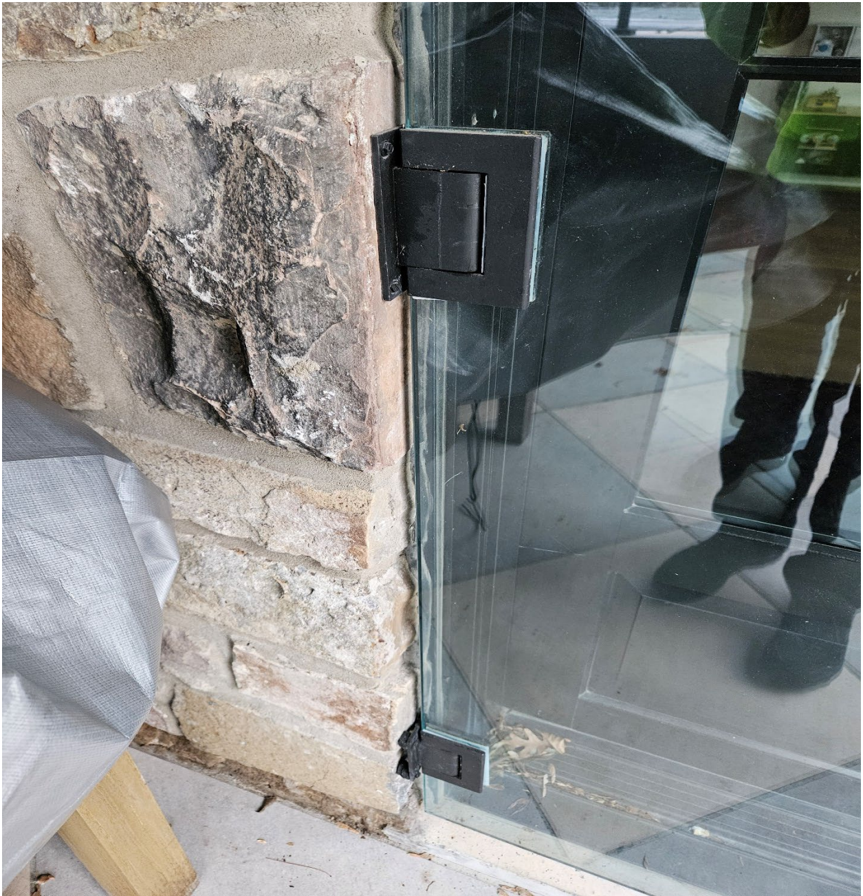
Attachment #4: Close up tempered glass gate mounted to exterior wall
