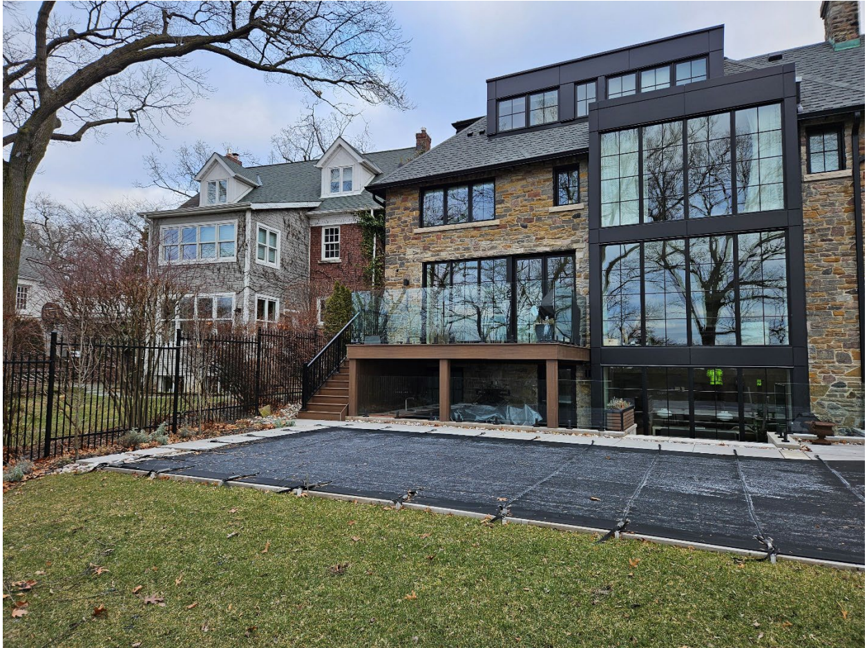
Attachment #1: View from rear yard facing dwelling
