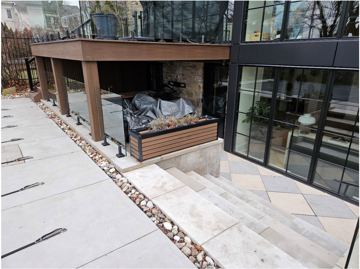
Attachment #2: View from pool deck facing basement walkout (gate)
