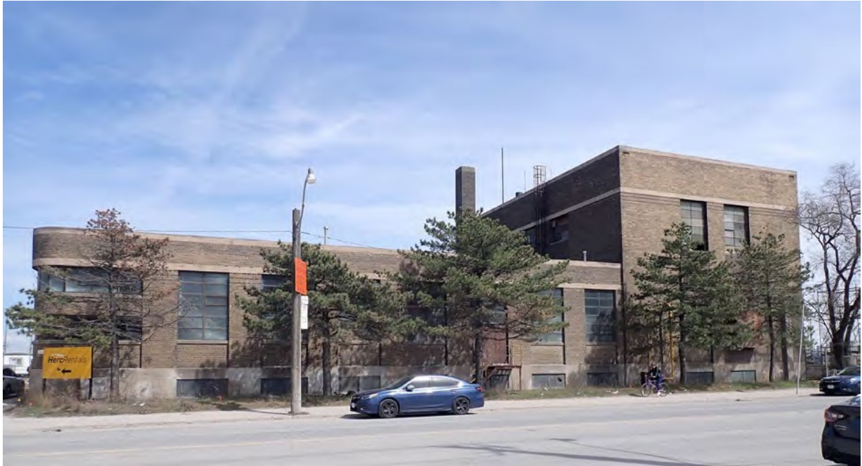
Canadian Oil Companies Ltd. Building - west elevation (source: HIA, ERA)
