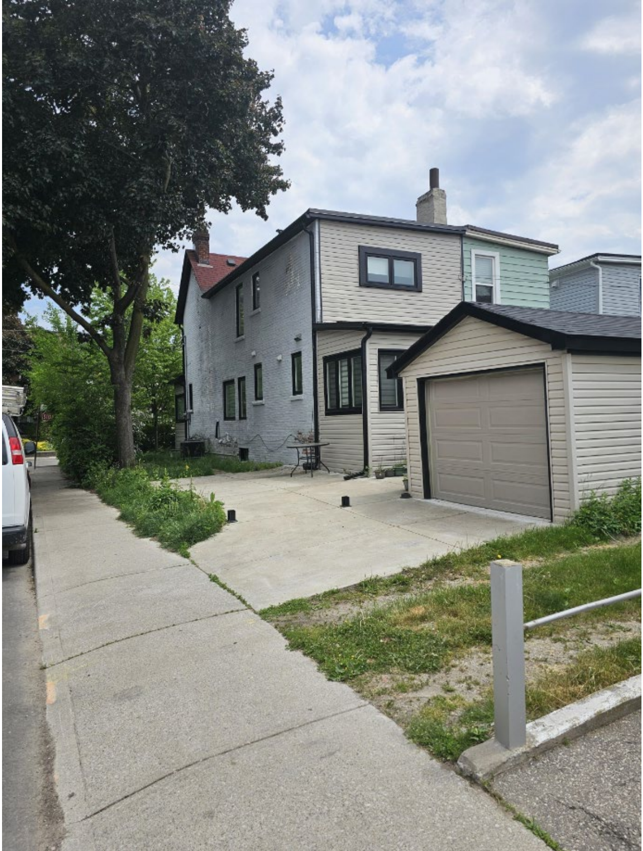
Attachment 3: Photo of the Shanly St flank of 308 Delaware Avenue
