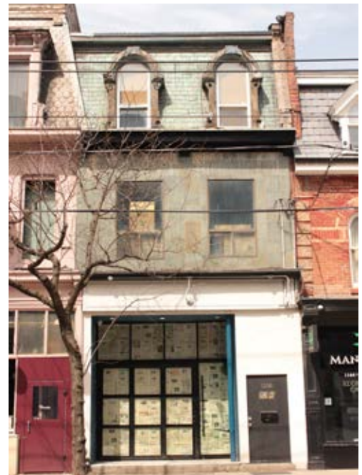
Figure 69: An over-clad building at 1166 Queen Street West whose historic building features may be restored with careful removal of the over-cladding.
