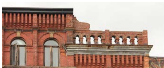
Figure 74: Detailed photo of the parapet at 660 and 664 Queen Street West that illustrates uneven repairs to deteriorated features but could be an opportunity for future restoration.
