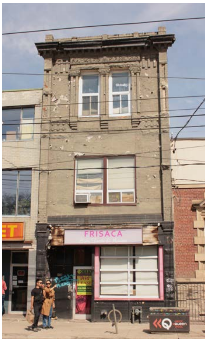
Figures 61, 62: Minimum standards for maintenance and occupancy of designated heritage properties are outlined in the City of Toronto Property Standards By-Law (top: 744-746 Queen Street West; bottom: 592 Queen Street West. Both properties exhibit areas of peeling paint, which may alternatively indicate or obfuscate further damage to the brick cladding underneath).
