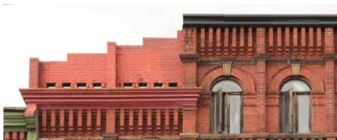
Figure 74: Detailed photo of the parapet at 660 and 664 Queen Street West that illustrates uneven repairs to deteriorated features but could be an opportunity for future restoration.
