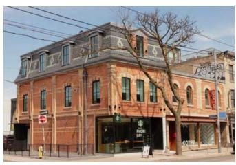
Figure 64: The same properties photographed in 2024, where the façade of 1026 Queen Street West has been restored and the polychromatic brick cladding of 1030 Queen Street West has been revealed.
