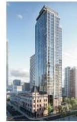
G. 8 Gloucester Street 34 Storeys (114m)
