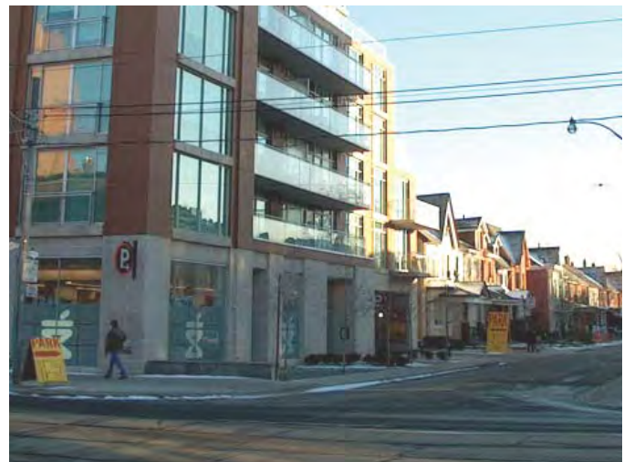
Illustration of a vehicular access point located off of a side streets.
