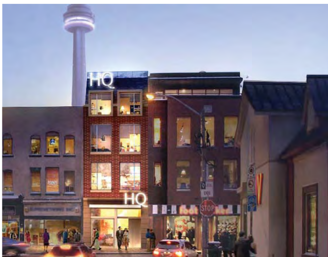
Three and four storey street wall. 8
