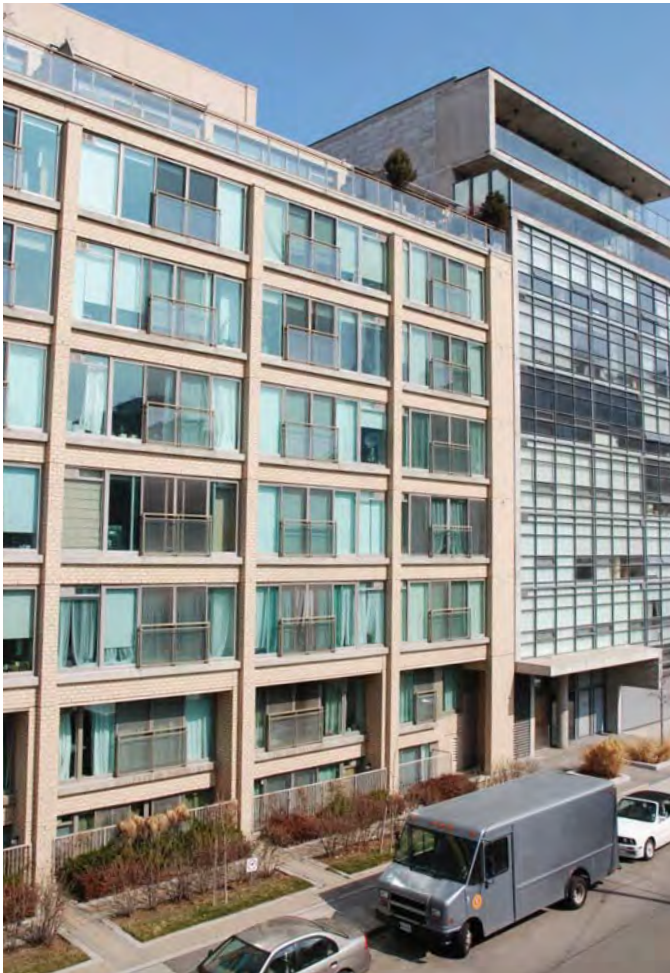
Continuous street wall.
