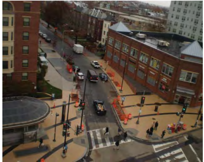
An example of a civic plaza framed by mid-rise buildings set back from the corner - Tivoli Square, Washington DC. 10,11
