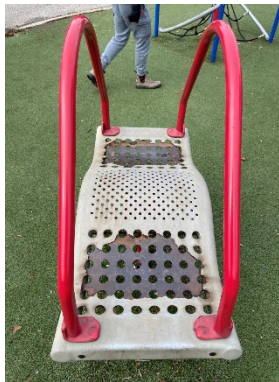
Photo 2: Large rust areas and surface coating lifting off playground equipment
