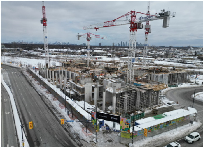
Bloor-Kipling Block 1 Construction
