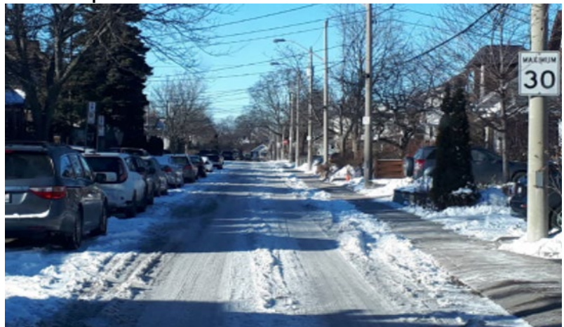
Example of Safe and Passable Pavement Conditions
