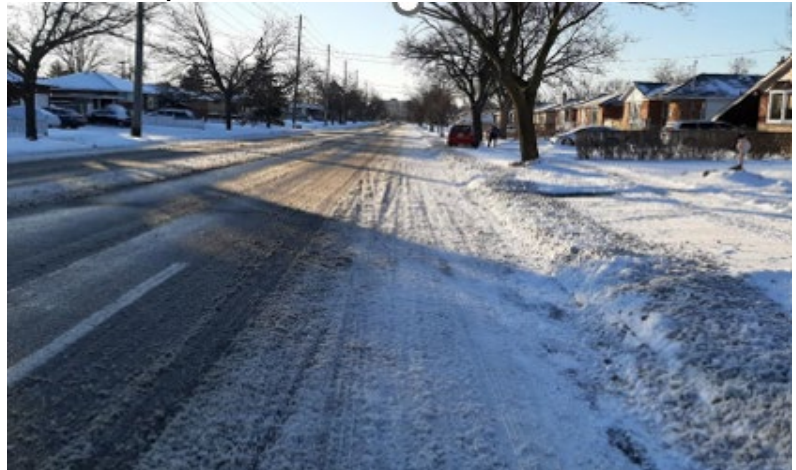
Example of Centre Bare Pavement Conditions
