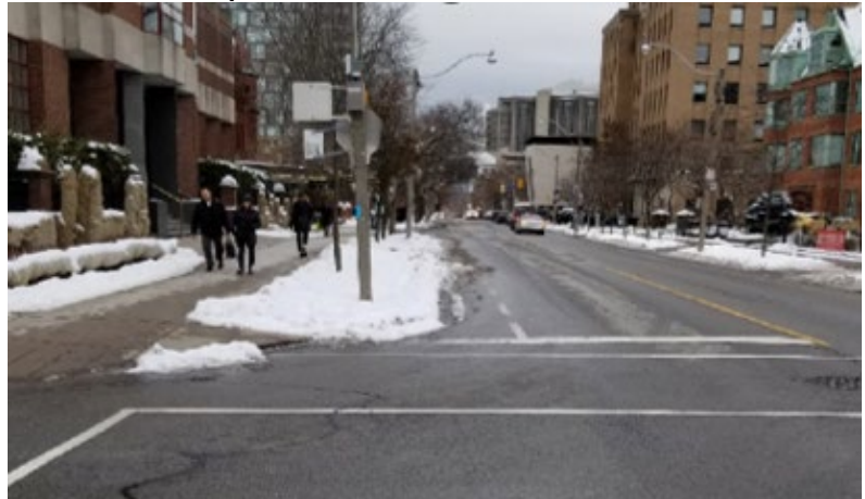
Example of Bare Pavement Conditions
