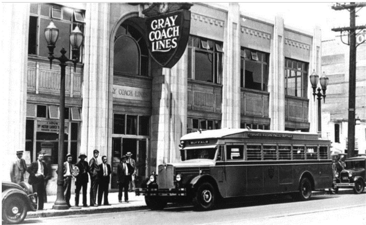
Figure 9: Archival photograph from July 1932, showing a detail of the cast aluminum spandrels and window mullion pattern. (City of Toronto Archives)
