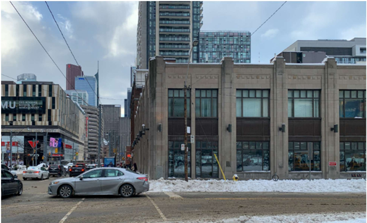
Figure 18: View south on Bay Street, from Edward Street. (Heritage Planning, 2025)
