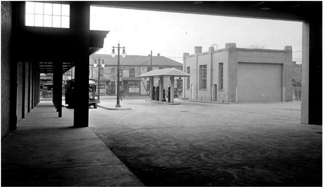
Figure 16: Archival photograph of the original bus yard, looking west. The covered arrivals platform is seen on the left side of the image and the inspection building and service platform (demolished) are seen on the right. (City of Toronto Archives)
