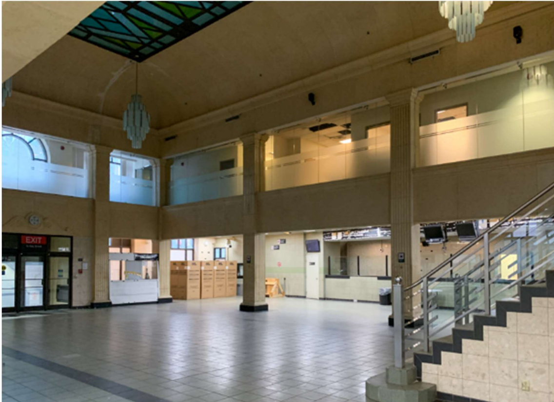
Figure 15: Current photograph of the terminal building entrance hall, looking southeast. (Heritage Planning, 2025)
