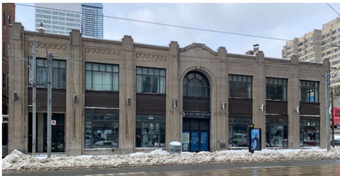
East (principal) elevation, former Gray Coach Terminal at 604 Bay Street, (Heritage Planning, 2025).
