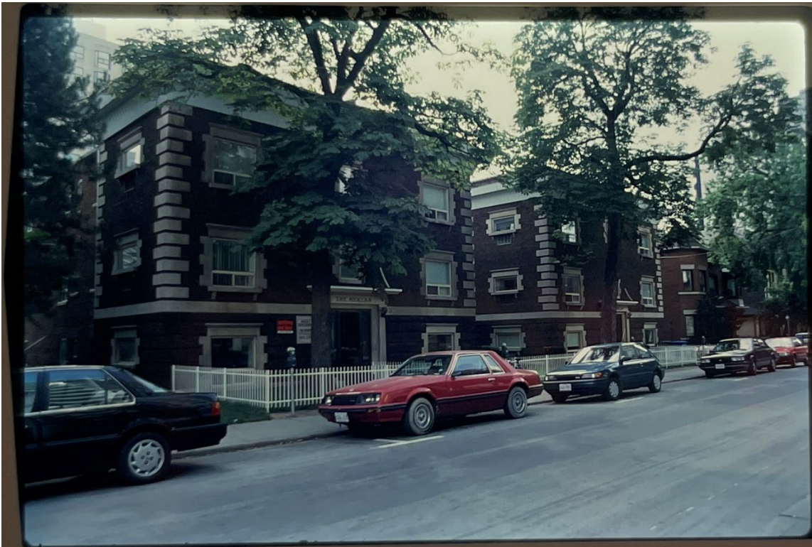
Figure 15. 1992 photograph of 81 Isabella Street, cornice and brick parapet have been over-clad (CTA).
