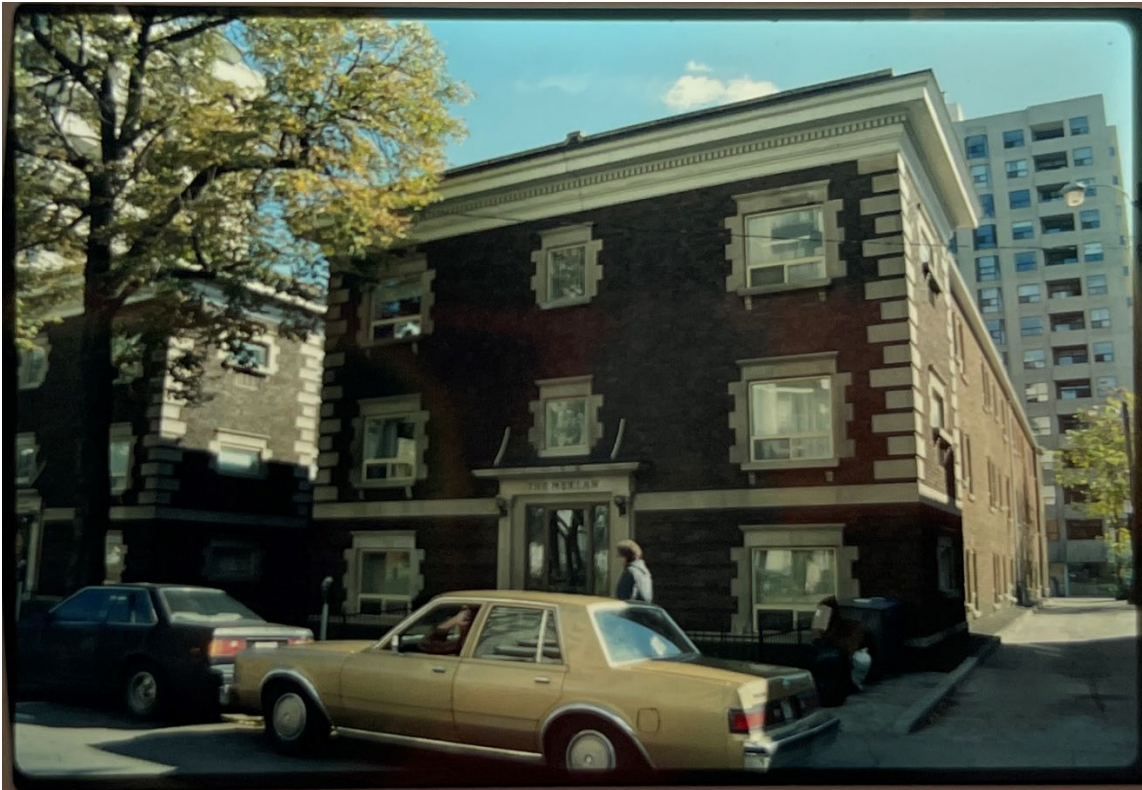
Figure 14. 1978 photograph of the western wing street-facing elevation at 81 Isabella Street, the cornice and brick parapet are visible (CTA).
