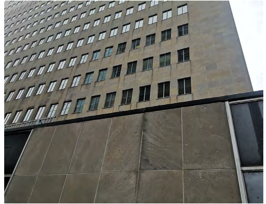
North elevation view, showing (at the bottom of the image) a portion of the one-storey volume with stone and granite cladding. Note the stone is in fair condition. Soiling is notable near the joints. Of note are some porous panels, which appears to be a natural imperfection of the stone and has not caused deterioration. On the north elevation of the tower, soiling below the window sills is noticeable at the corners, due to a lack of proper edge detailing.
