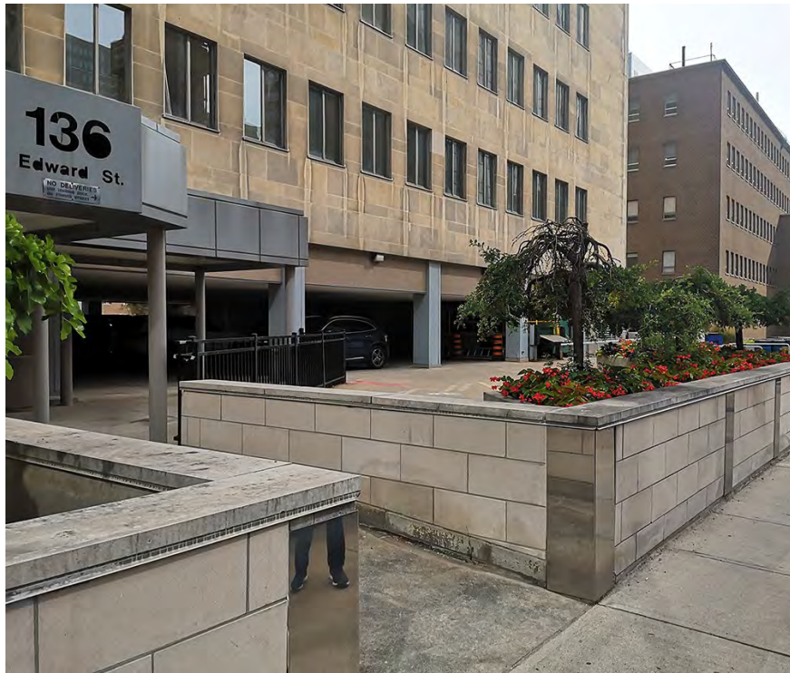
Looking east on Edward Street, showing the bottom portion of the south elevation that is set back from Edward Street. The parking garage is at grade and located underneath the second storey of the building. This parking is hidden by the one-storey base volume (not visible in the photo). The low-rise stone barriers in the foreground are later additions. Note similar conditions of the stone to that found on the north elevation, with soiling evident at the bottom of the sills.
