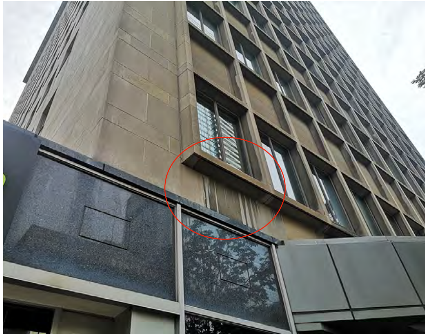
Close-up view of the west elevation, looking up towards fenestration pattern. Drip edges carved into the underside of the stone sills are visible and were added to deflect water away from the walls. These appear to have worked on all areas below window sills. Below the window sill of the bottom left window (red circle), some water run-off is visible, suggesting a potential issue in this area. This is associated with the wall section from the previous page where the stone cladding meets the granite cladding below. However, in the current condition, the granite is not in the same plane as the stone (it is in front of the stone) which differs from the 1956 drawing, suggesting a potential difference in the backing of the granite cladding.
