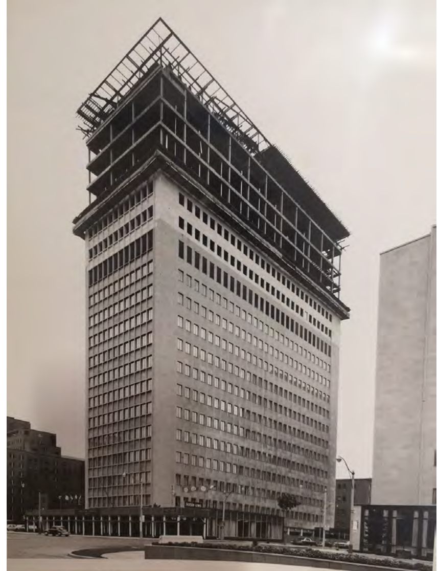
Under-construction addition. Note the two storeys above the mechanical floor (noticeable by the taller window openings) are visually different (Source: CTA).
