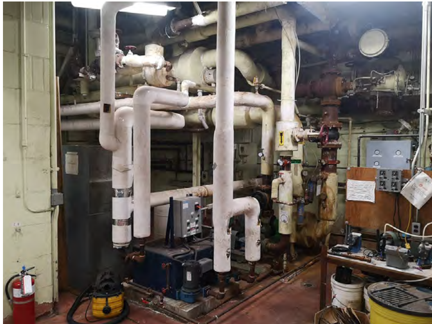
Overall view of original mechanical equipment (heat pumps). The partition walls on the left of the photo are painted hollow terra cotta tiles.
