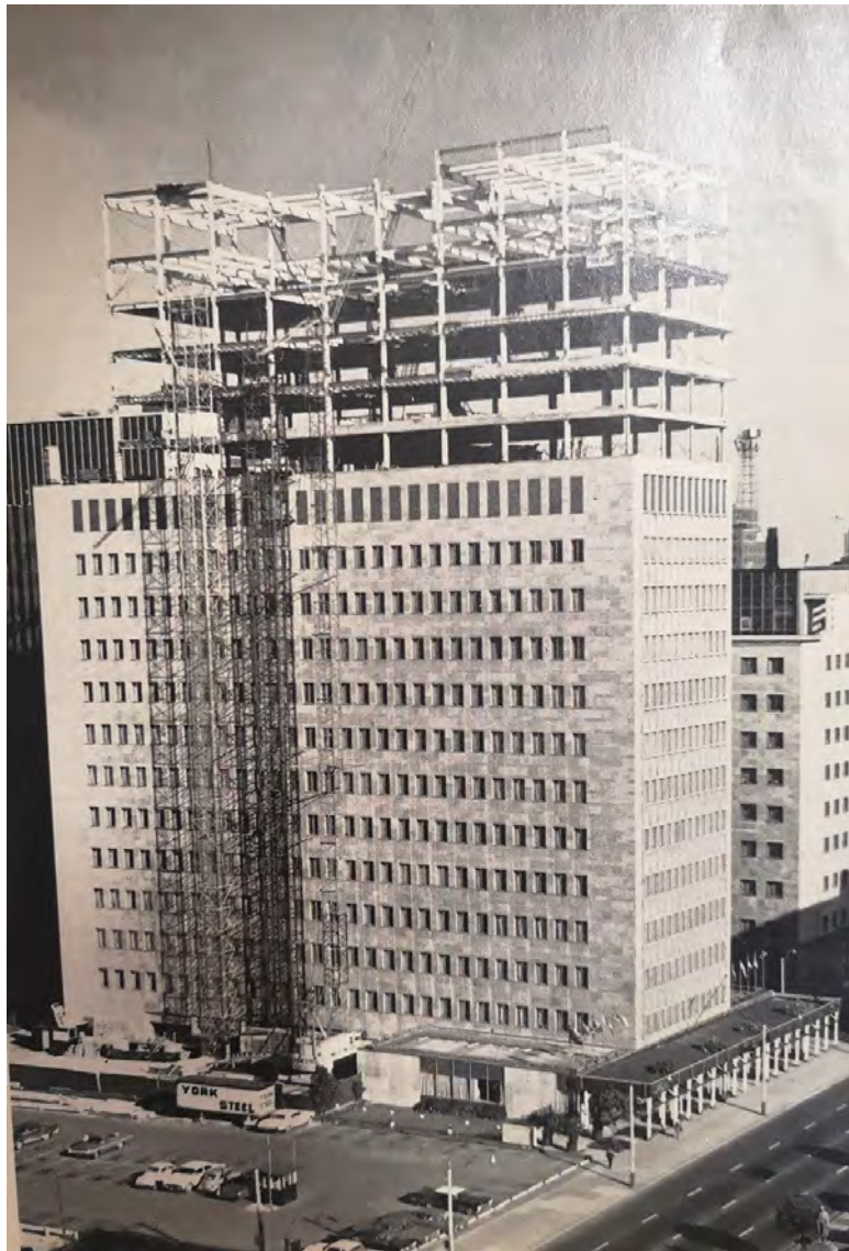
Under-construction addition , showing the north elevation and the crane used to hoist the steel to the new upper storeys (Source: CTA - Engineering and Contract Record, December 1965).
