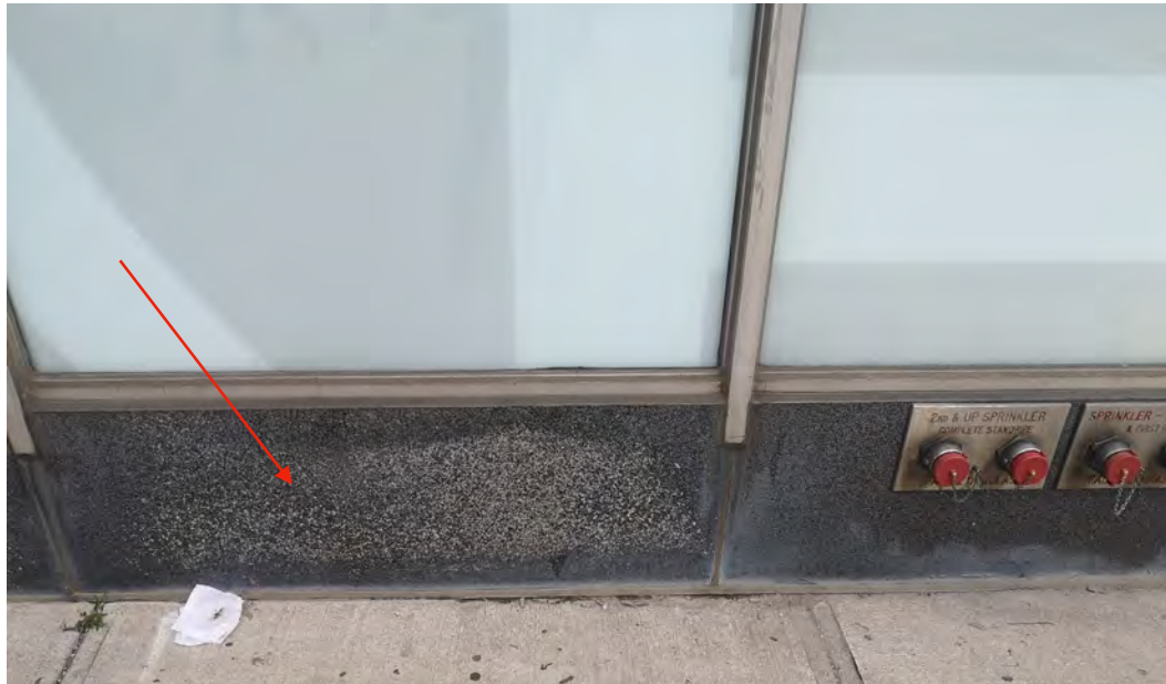
Lower portion of the one-storey volume, facing University Avenue, showing a discoloured granite panel (arrow).
