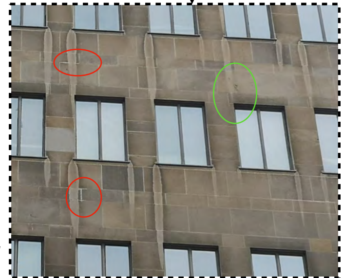
Looking towards the overall south elevation and the consistent soiling below the sills. Localized areas of mortar repointing appear to have been inappropriately completed (red circle) and some localized panels appear to be damaged (green circle)
