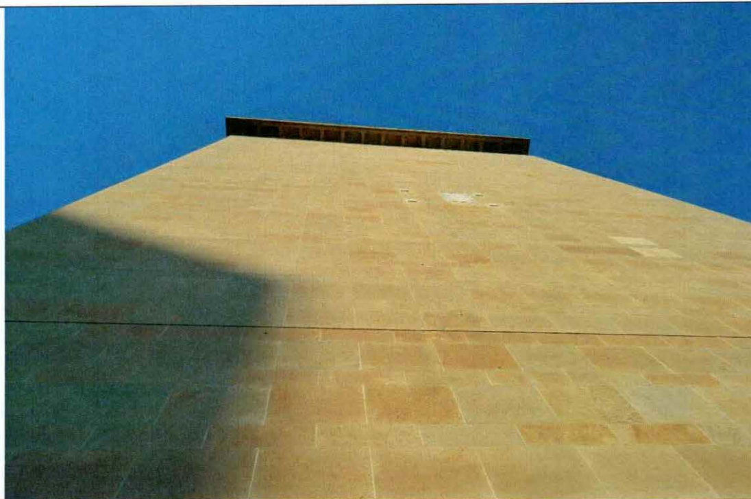
Figure 61 East elevation floors 12-20. The masonry is in good condition.
