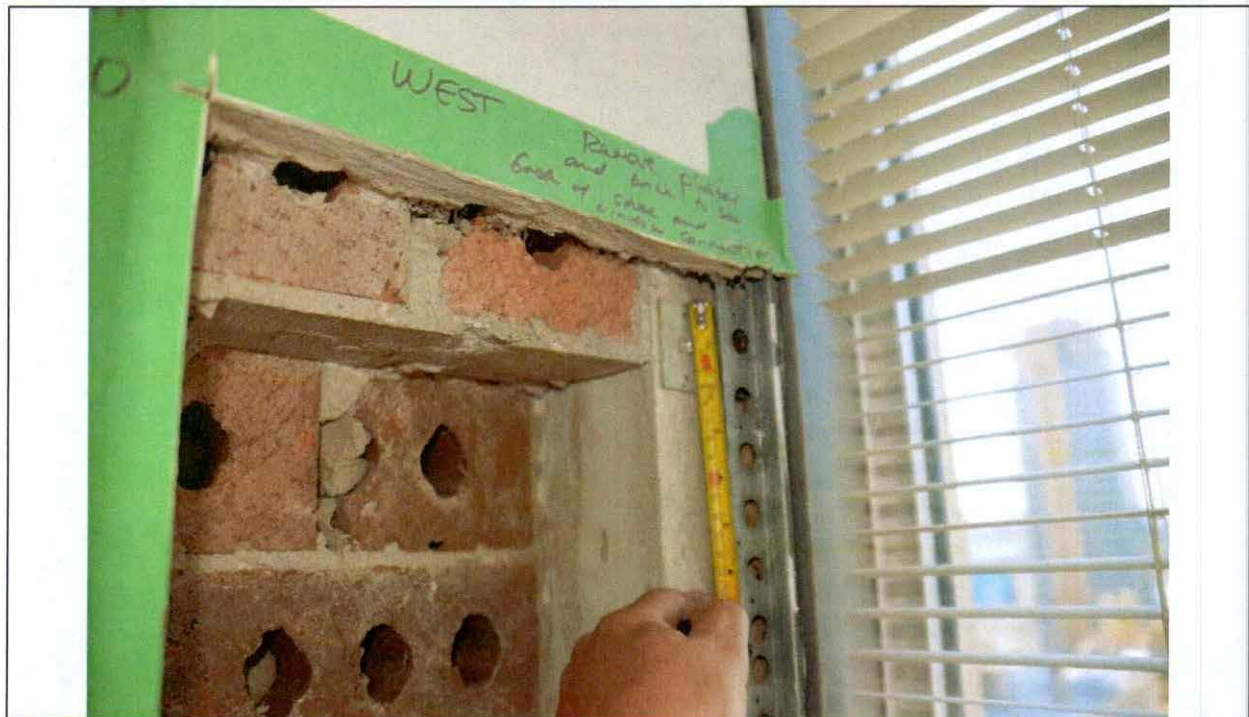
Figure 29 Investigation opening #10 Detail. Stone window reveal mullion with brick backup. Window tie anchored with #12 Galvanized screw. No moisture barrier was found.
