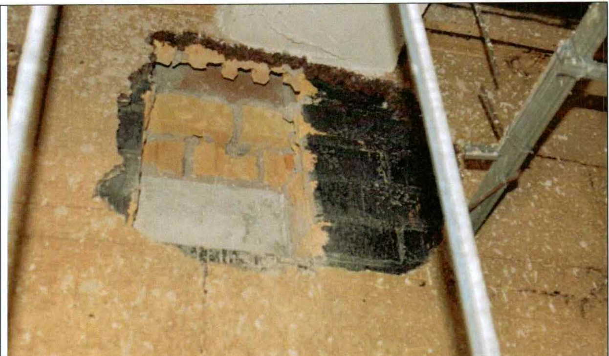
Figure 45 Investigation opening #18 Detail. Corkboard and brick masonry were removed. Stone is block bonded into backup.
