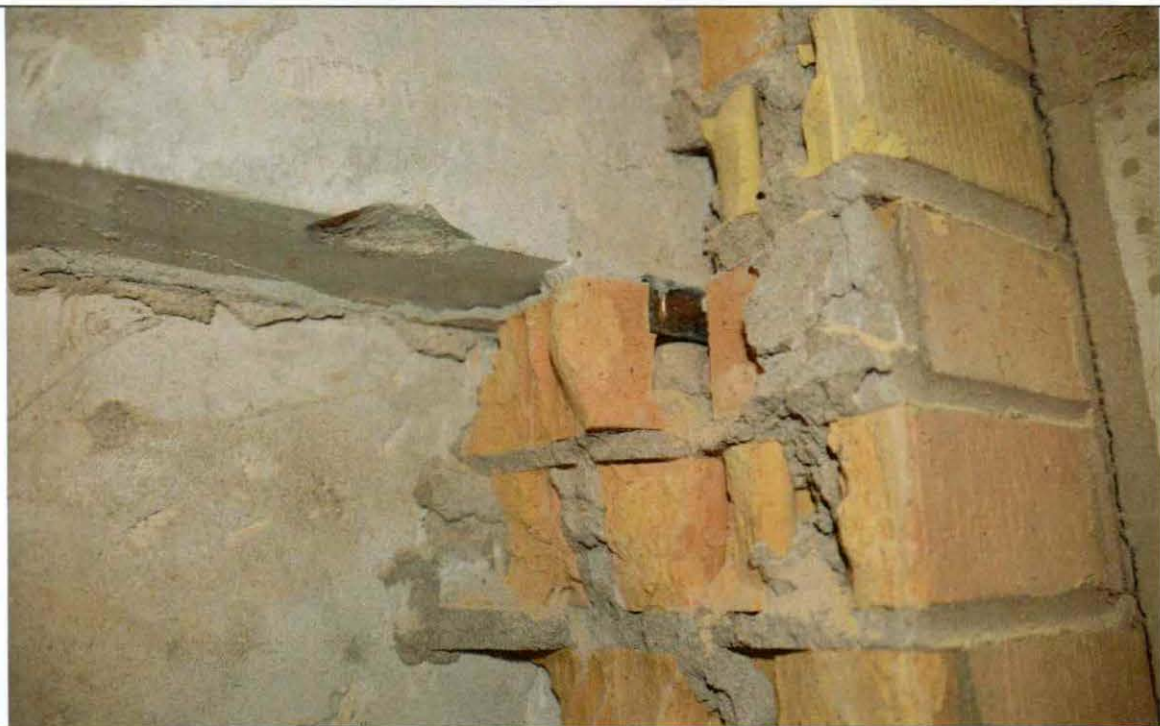
Figure 31 Investigation opening #11 Detail. Stone veneer is block bonded with brick backup. One bronze wall tie was found (RHS).
