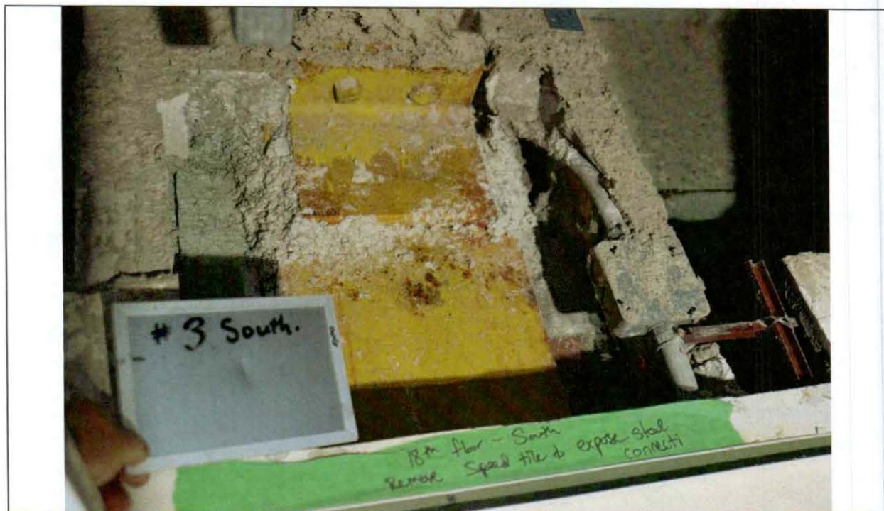
Figure 14 Investigation opening #3 at column and beam connection Fire protection was removed.
