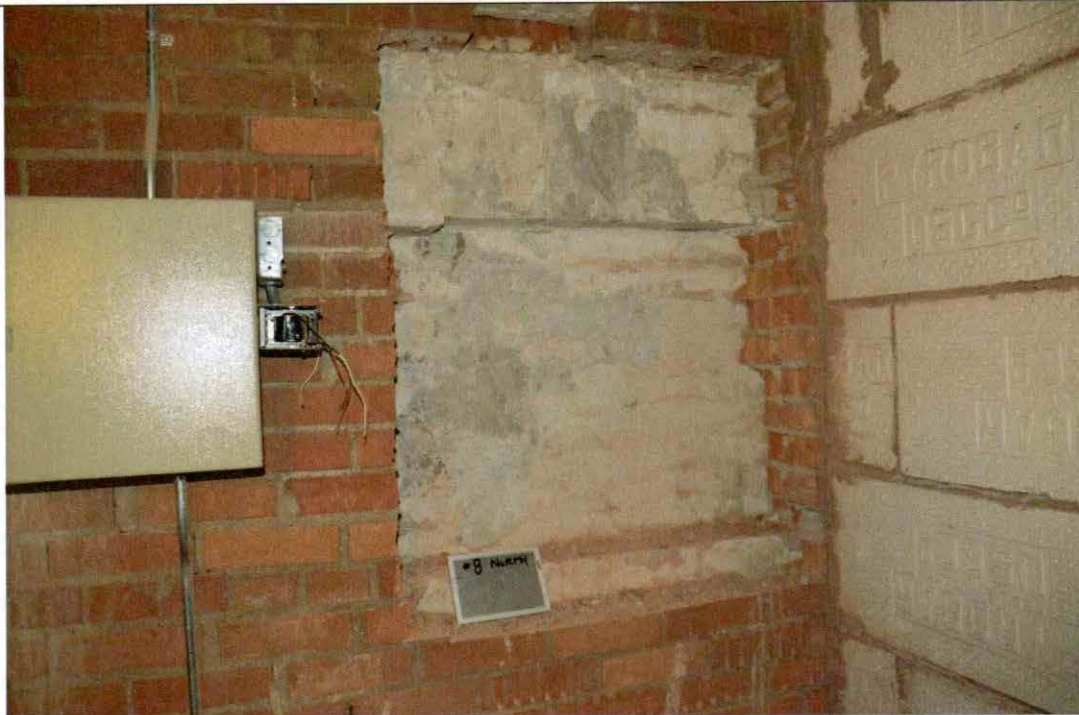
Figure 24 Investigation opening #8 in vent shaft.
