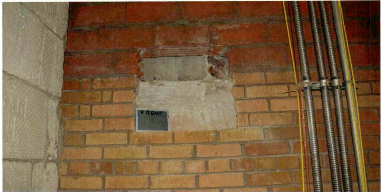
Figure 32 Investigation opening #12 in vent shaft.
