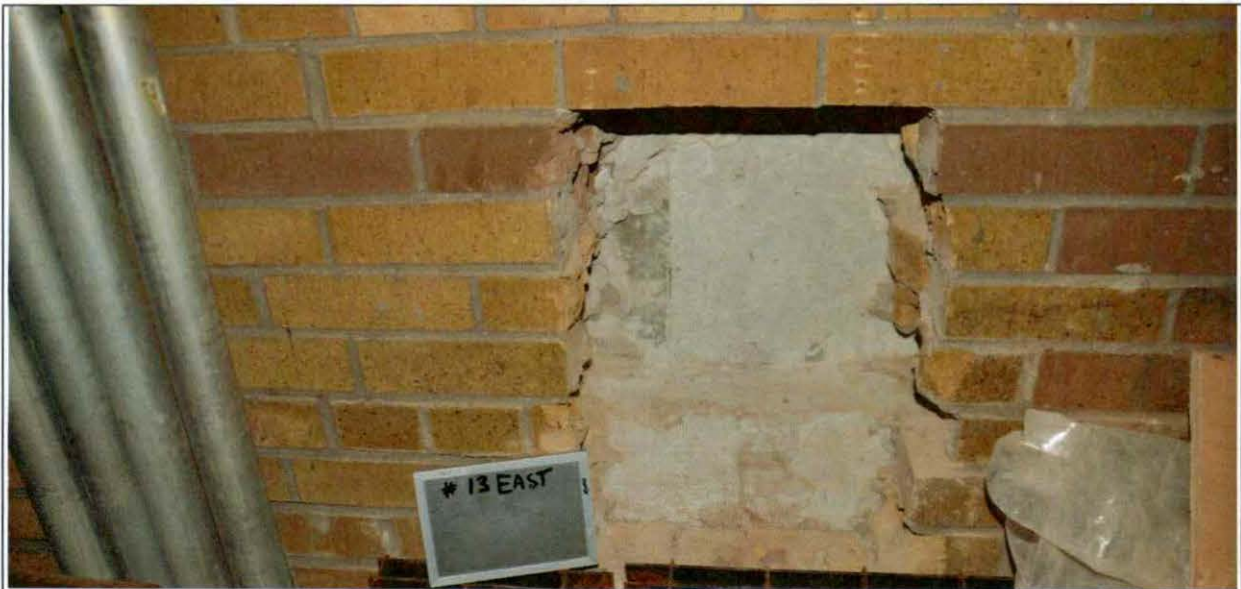
Figure 34 Investigation opening #13 in vent shaft.
