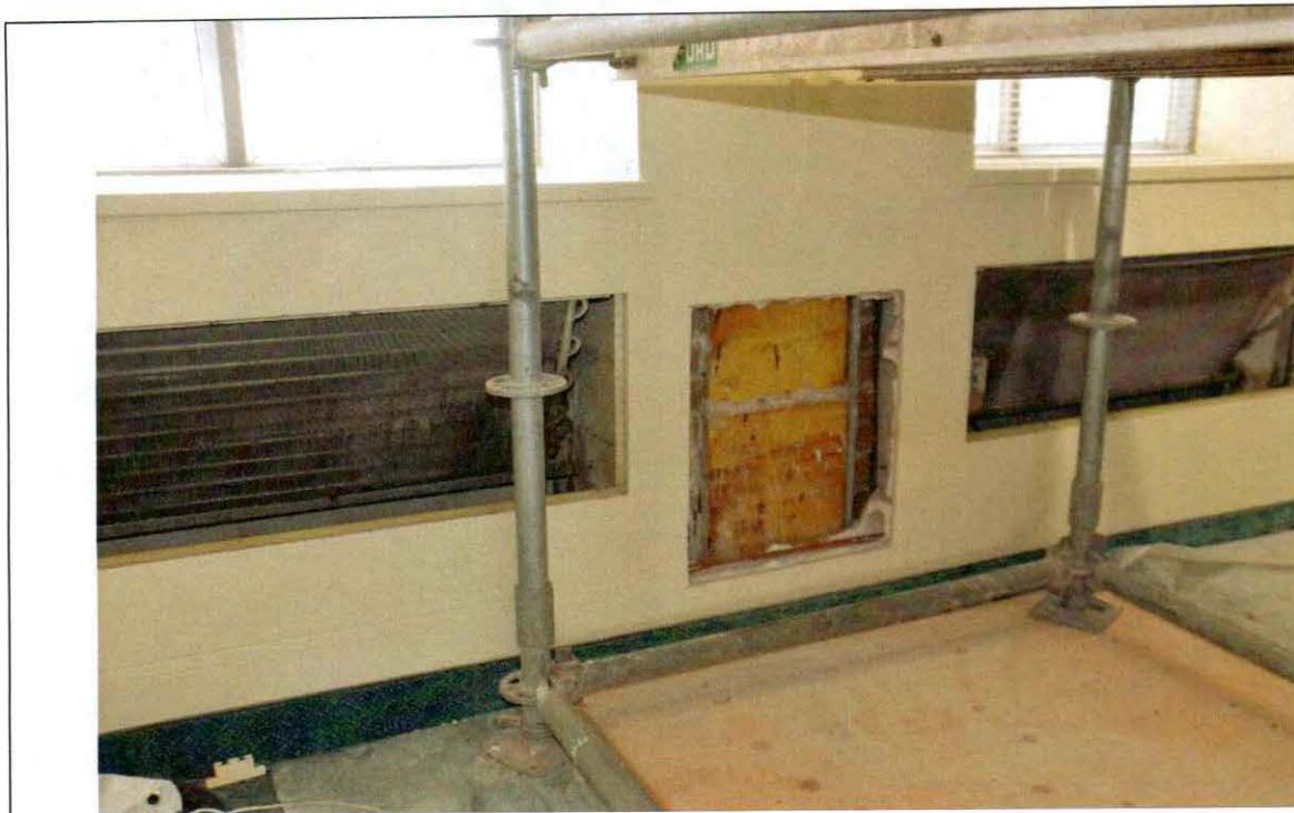
Figure 12 Investigation opening #2 at column location.
