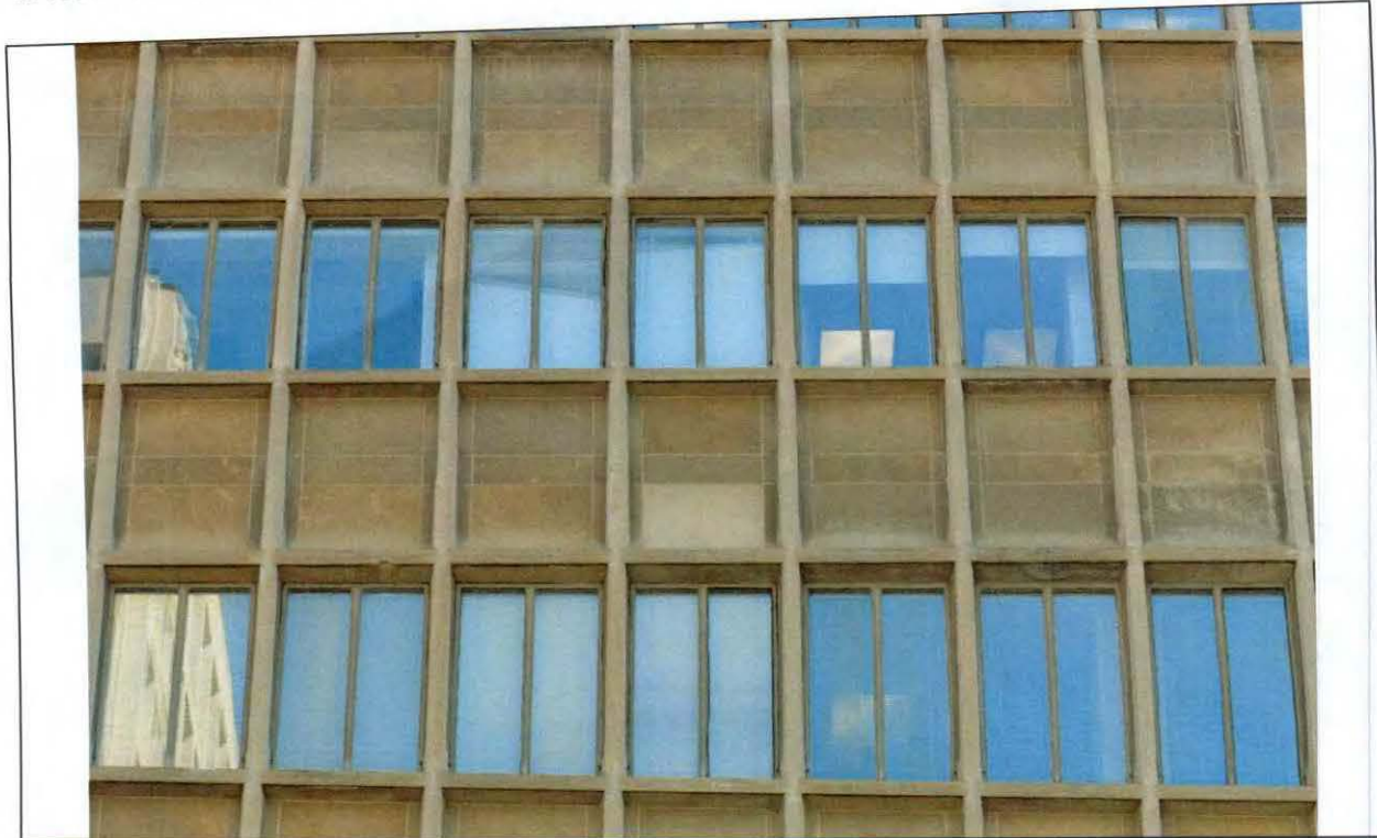
Figure 84 West elevation lost section of drip edge on lintel and typical sill/ lintel weathering erosion at the 4-5 th floors.
