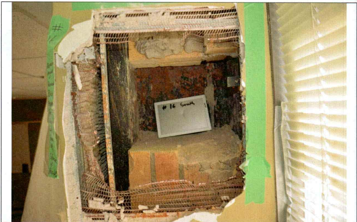
Figure 41 Investigation opening #16 Detail. The brick infill was removed. Some coating failure on steel and light corrosion are evident (black paint).
