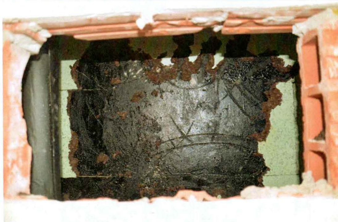
Figure 51 Investigation opening #21 Detail. The corkboard was removed back of the stone was parged and bitumen paint coated.
