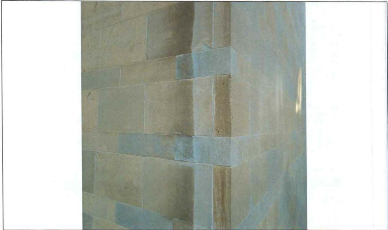
Figure 58 Southeast corner elevation at the 2 nd floor. Note that debonded joints continue to grade.
