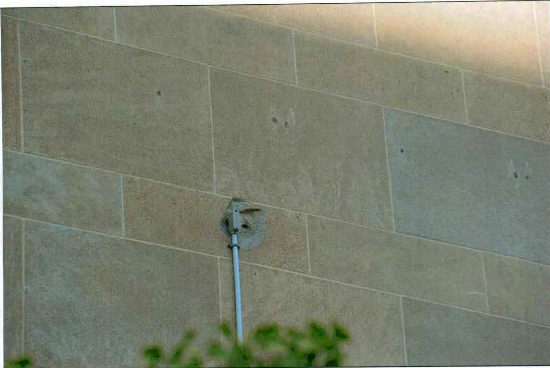
Figure 60 South elevation-west side spalled stone at electrical service penetration and holes in cladding from fixings.
