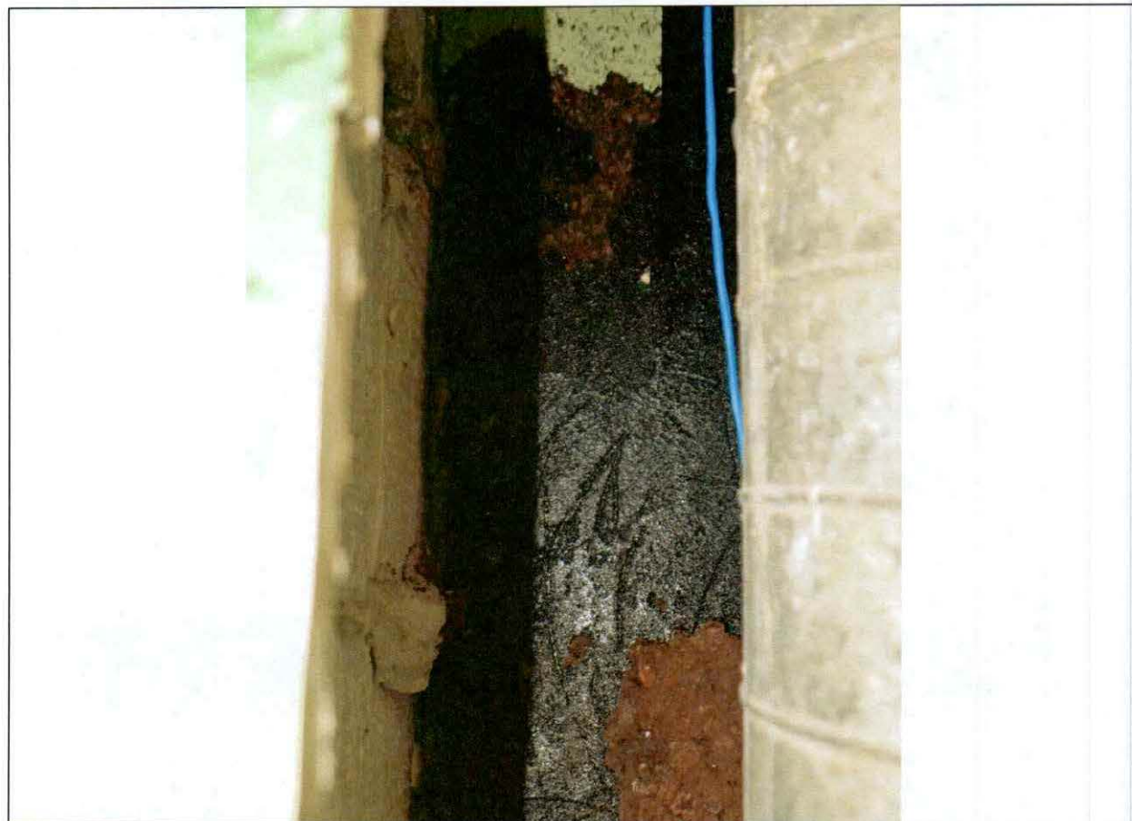
Figure 17 Investigation opening #4 Detail. The corkboard insulation was removed. A bituminous layer over parged stone masonry was found.
