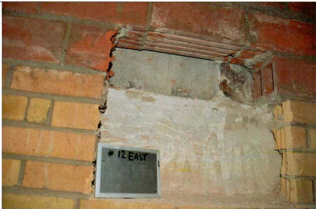
Figure 33 Investigation opening #12 in vent shaft Detail. Stone veneer with brick backup- replaced Indiana limestone (vent infill) at upper. No ties were found.
