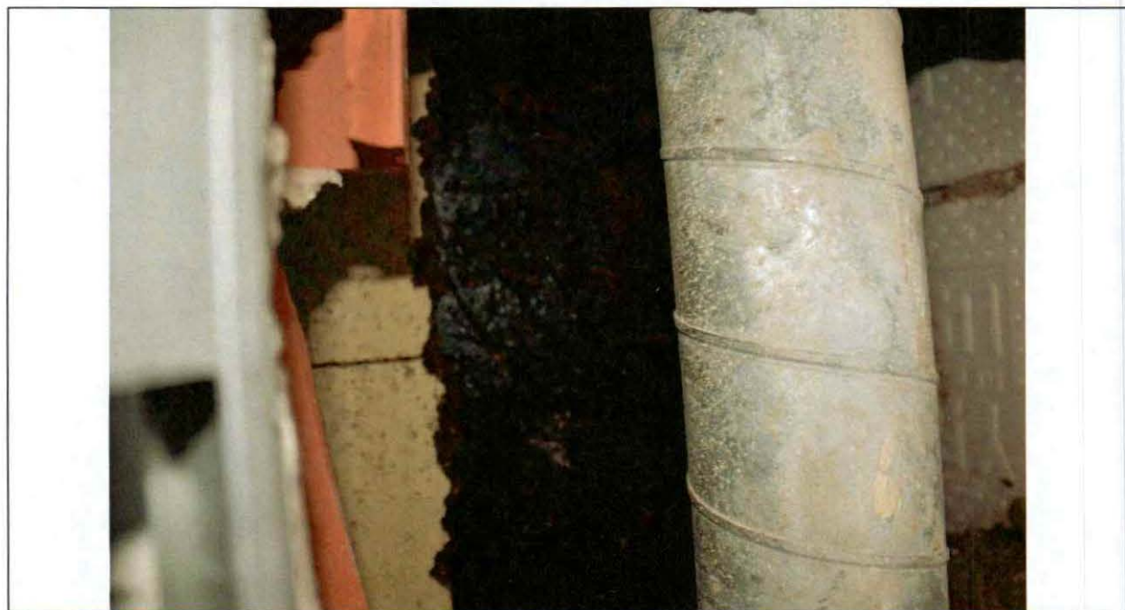
Figure 27 Investigation opening #9 Detail. The corkboard insulation was removed. A bituminous layer over parged stone masonry was found.
