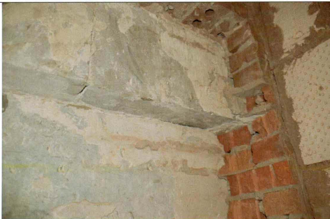
Figure 25 Investigation opening #8 Detail. Stone veneer is block bonded with brick backup. No ties were found.
