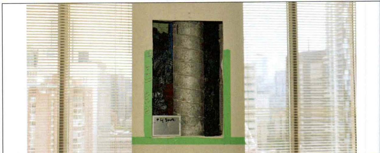
Figure 16 Investigation opening #4 spiral vent duct in front of mullion masonry
