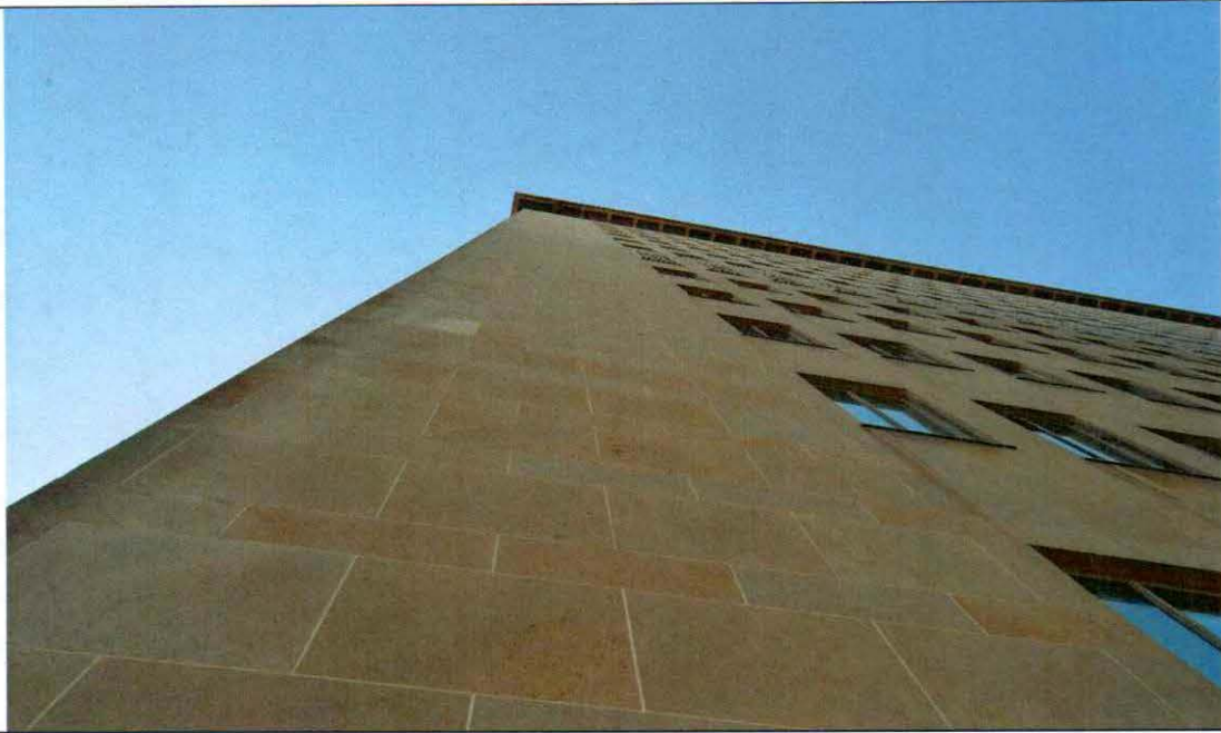
Figure 66 North elevation at east end floors 8-20. The masonry is in good condition.
