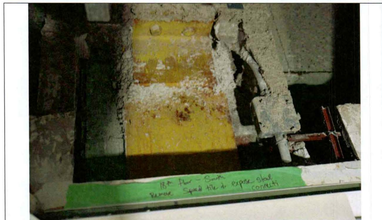
Figure 15 Investigation opening #3 Detail. The paint coating is in good condition.
