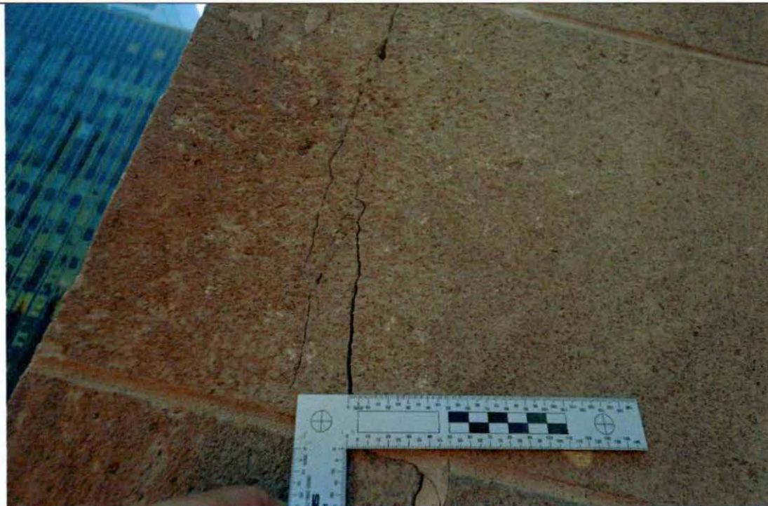
Figure 71 North elevation northeast corner. Detail of Crack/ displacement at 3 rd floor.
