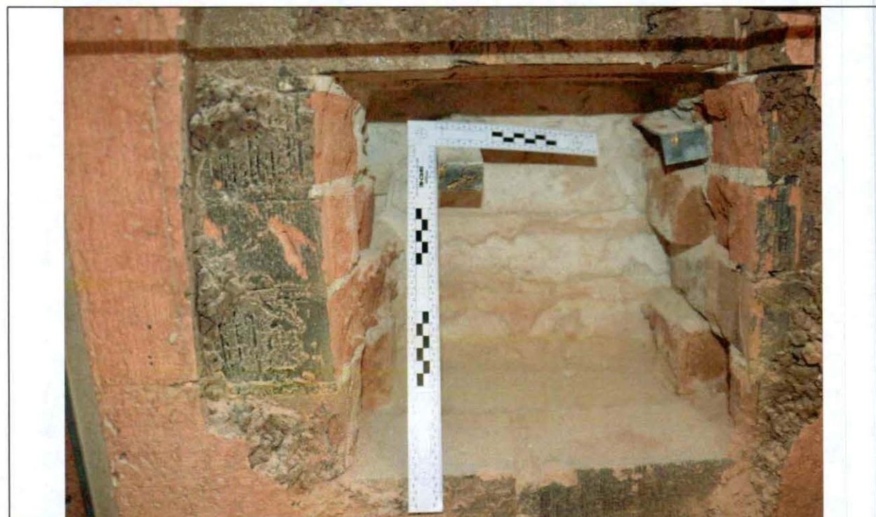
Figure 39 Investigation opening #15 Detail. Corkboard and brick masonry were removed. 2 ties were found- ties appear to be bronze (or similar copper alloy) and in good condition.
