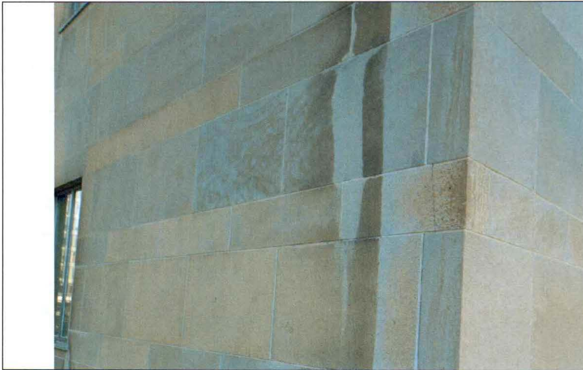
Figure 56 Southeast corner elevation at 4 th floor. Note cracked stone and debonded joints.
