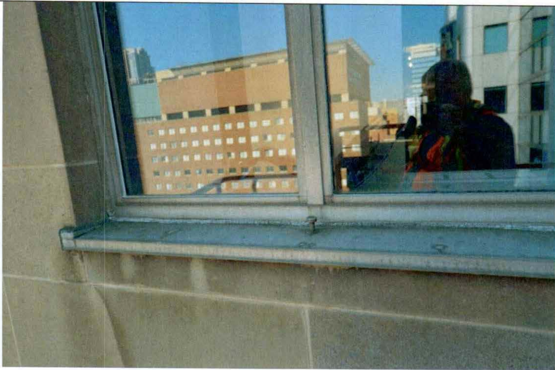
Figure 76 North elevation typical window condition- sealants failing and window frames heavily oxidized.
