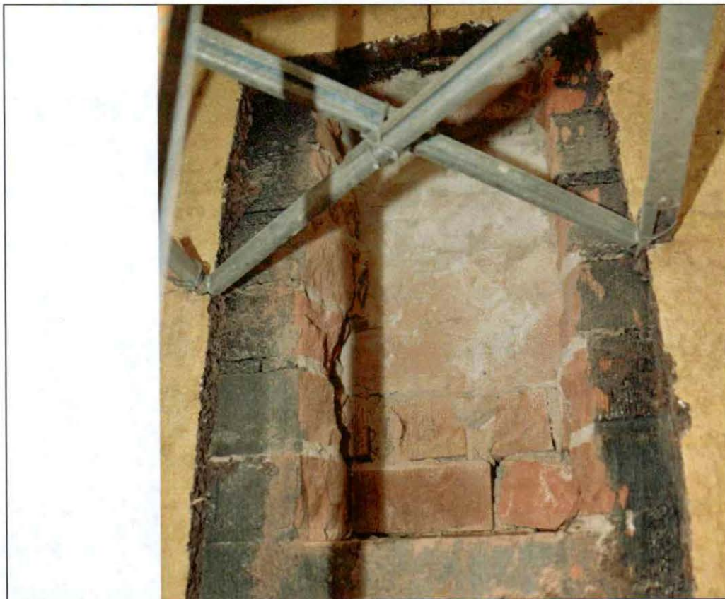
Figure 47 Investigation opening #19 Detail. Corkboard and brick masonry were removed. Stone is block bonded into backup.
