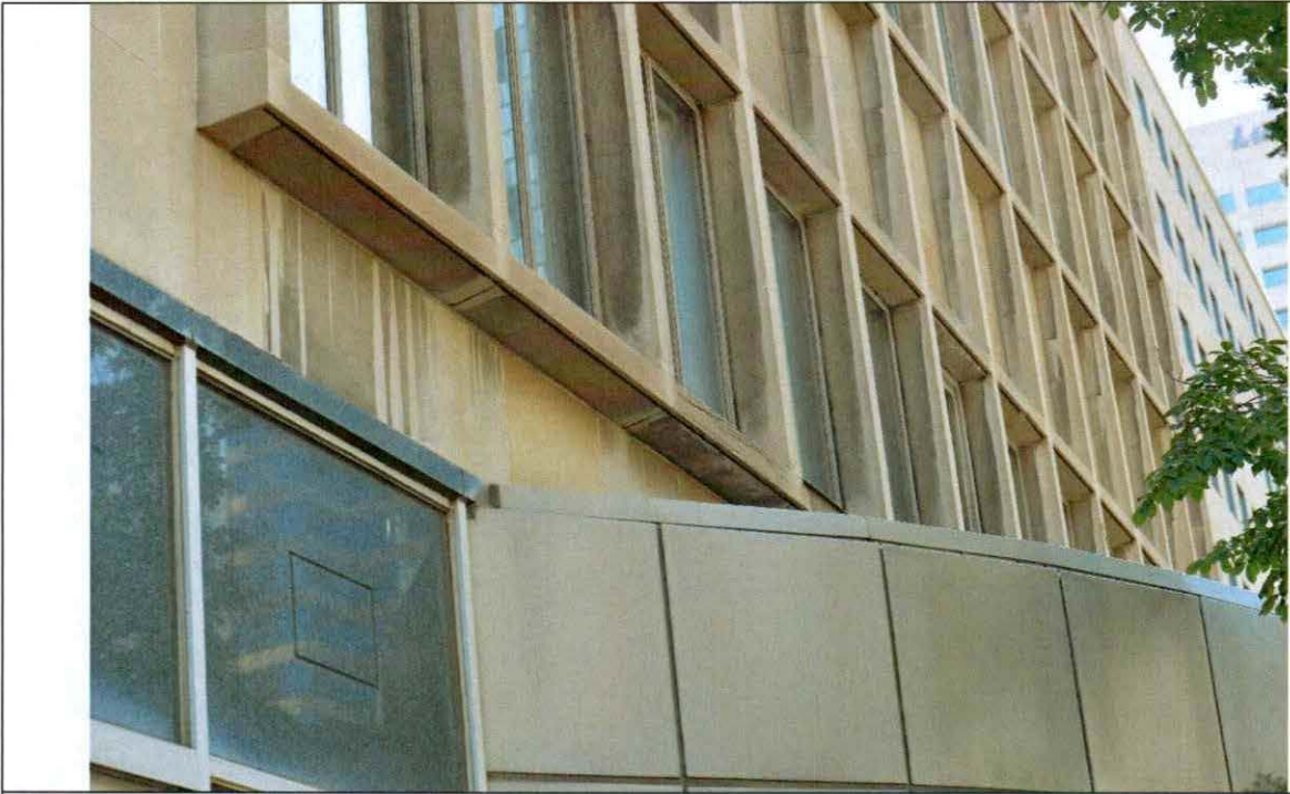
Figure 78 West elevation eroded sill at the 2 nd floor window.
