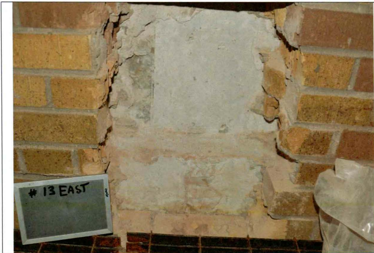
Figure 35 Investigation opening #13 in vent shaft Detail. Stone veneer is block bonded with brick backup. No ties were found.
