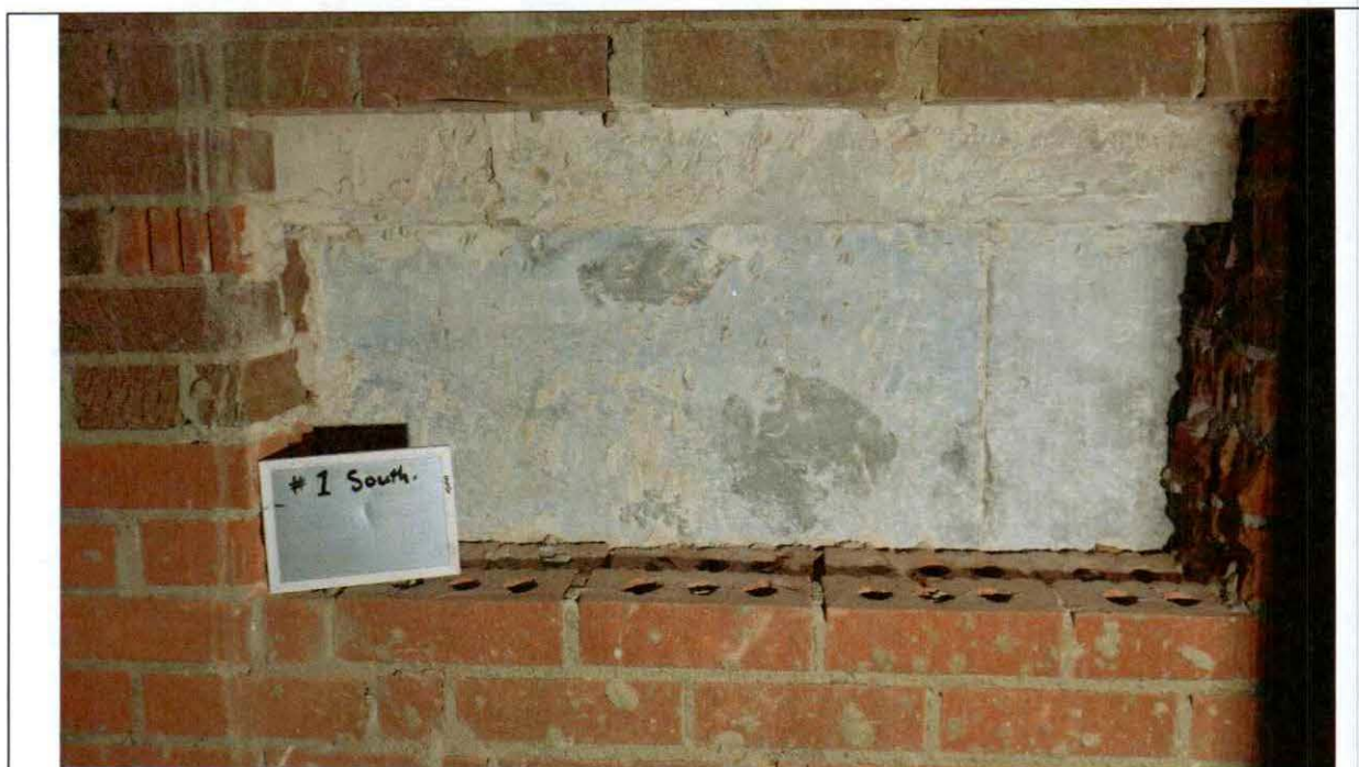
Figure 10 Investigation opening #1 in vent shaft. 2 wythes brick masonry to back of stone.
