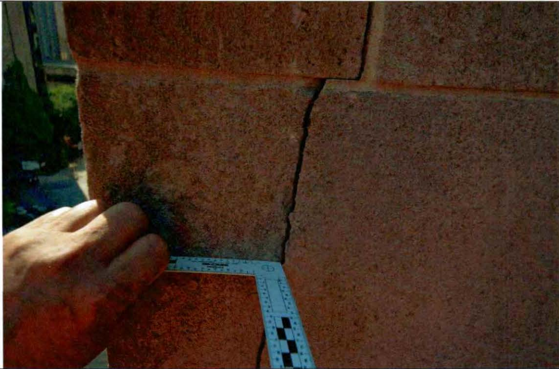
Figure 70 North elevation northeast corner. Detail of Crack/ displacement at 4 th floor.
