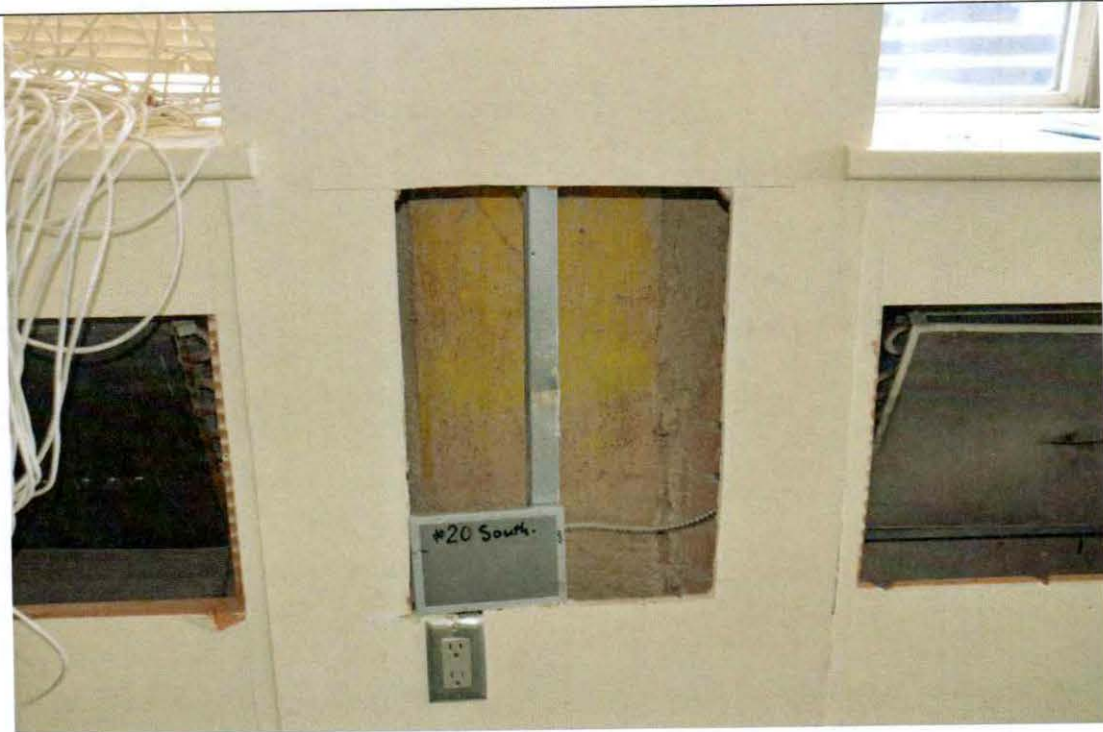
Figure 48 Investigation opening #20 at column.
