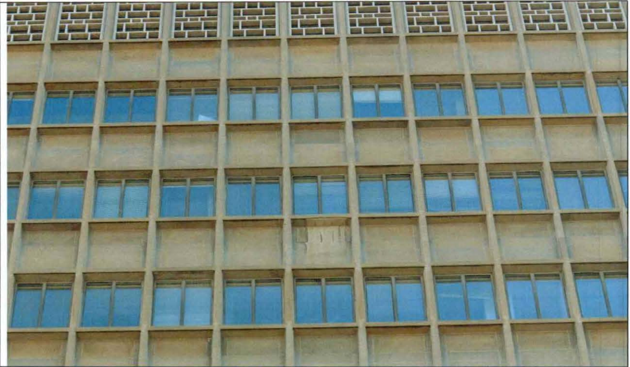
Figure 82 West elevation lost section of drip edge on the sill at the 11 th floor.
