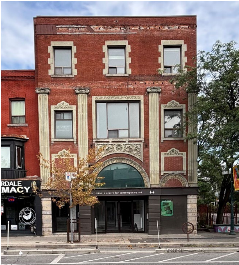
1286 Bloor Street West, south elevation (Heritage Planning, 2025).
