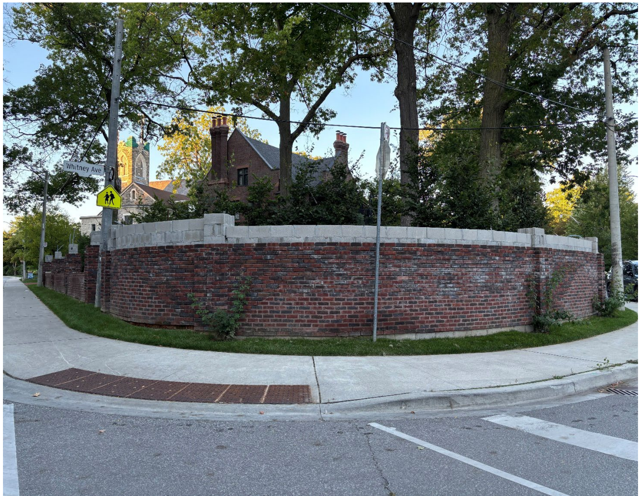
Contextual view of wall structure requested in the permit application looking northeast towards 2 Whitney Avenue from the corner of Glen Road and Whitney Avenue (City of Toronto, August 2025)
