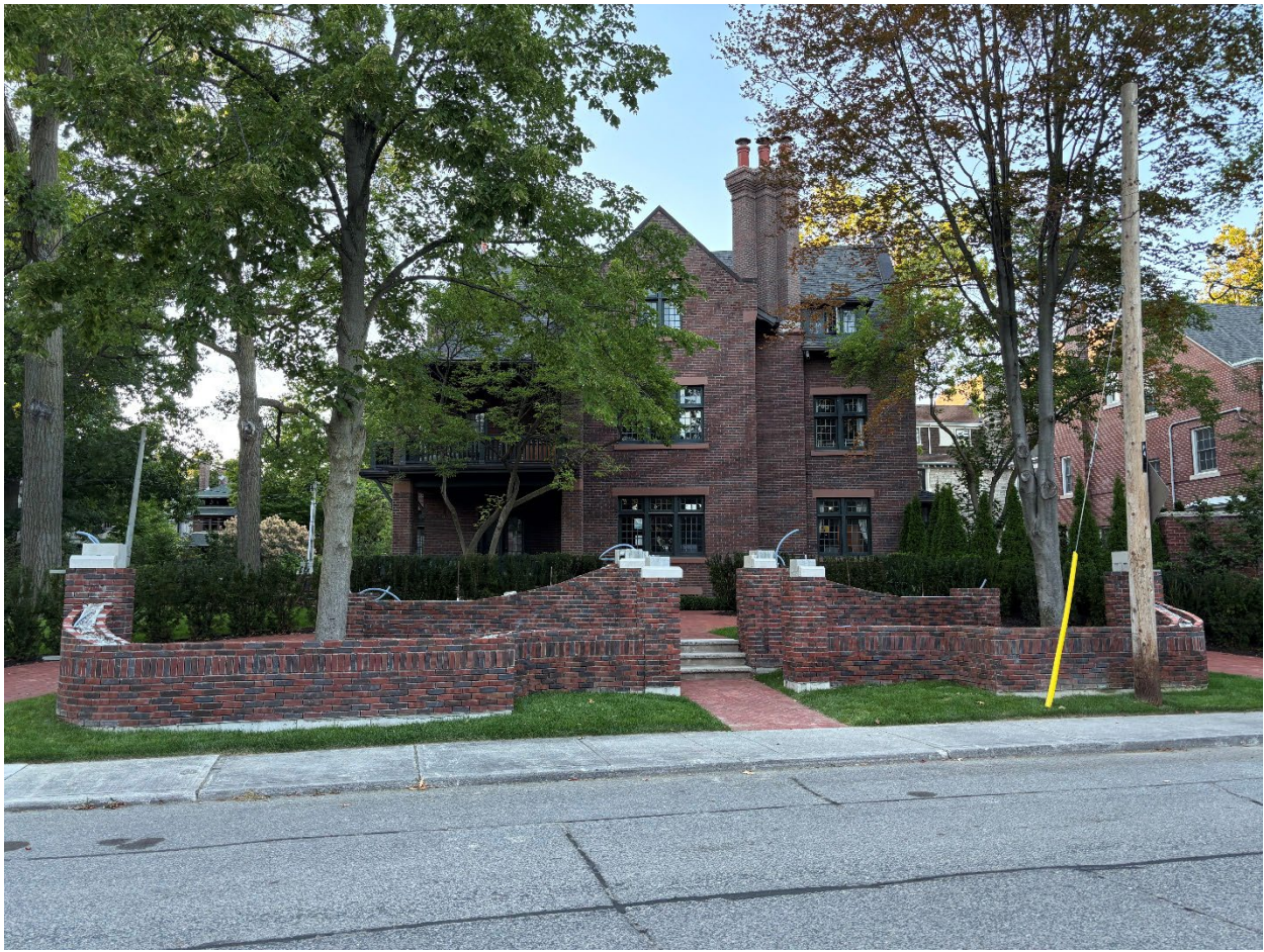
Contextual view of wall structure requested in the permit application looking south towards 2 Whitney Avenue from Whitney Avenue (City of Toronto, August 2025)
