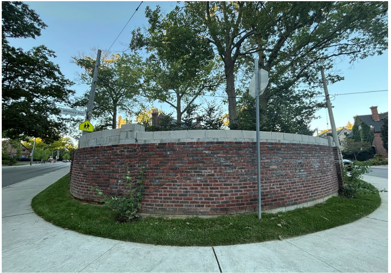
Detailed view of wall structure requested in the permit application looking northeast towards 2 Whitney Avenue from corner of Glen Road and Whitney Avenue (City of Toronto, August 2025)
