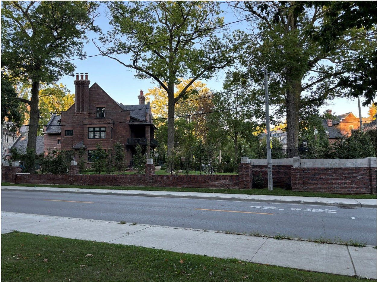
View of wall structure requested in the permit application looking east toward 2 Whitney Avenue from Glen Road (City of Toronto, August 2025)
