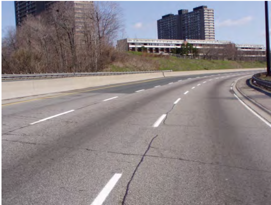
Figure 1-7 Example of Expressway in Poor Condition. Presence of intermittent to frequent cracks, rutting and distortions. Road surface is uneven and rough to drive.
