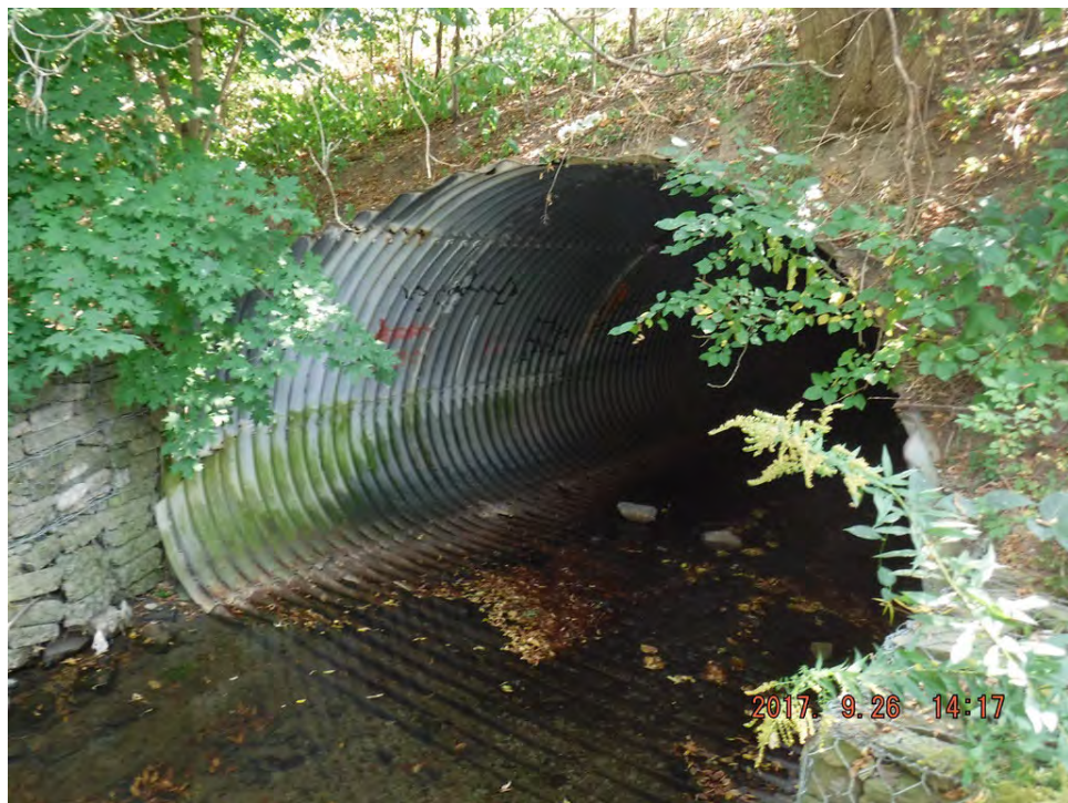
Figure 1-19 Example of a Culvert in Poor Condition - ID 267 Albion Rd over Albion Creek.
