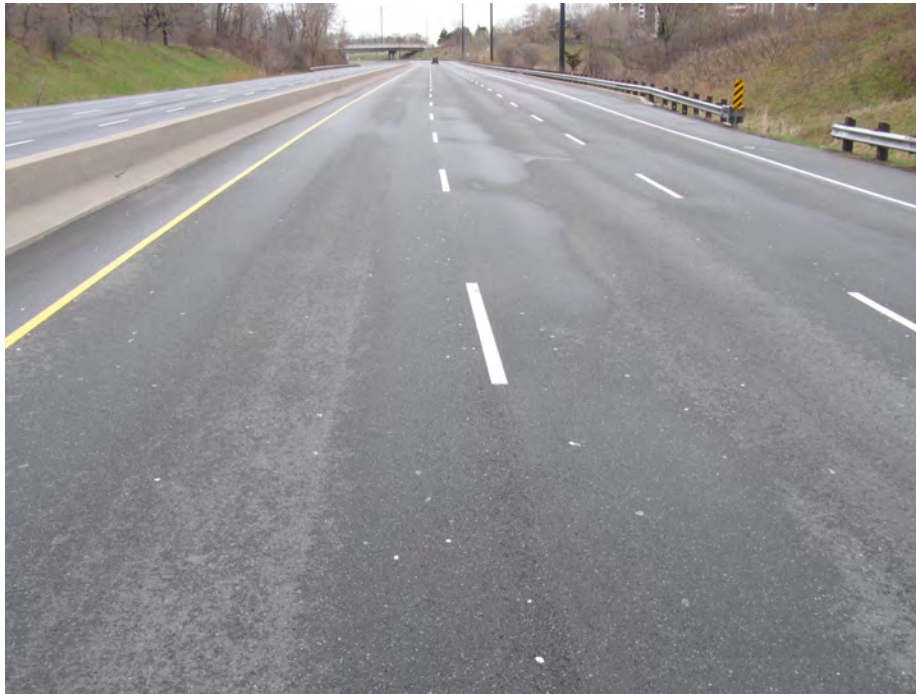
Figure 1-5 Example of Expressway in Good Condition. Road surface recently repaved and there are no cracks or surface deformations.
