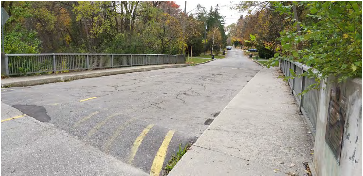
Figure 1-16 Example of a Bridge in Poor Condition - ID 758 Don River Blvd over Don River.
