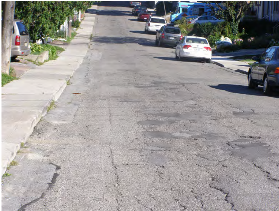
Figure 1-13 Example of a Local Road in Poor Condition - potential reconstruction candidate as overall pavement structurally failed. Presence of extensive alligator cracks, settlements and distortions. Road surface is very uneven and rough to drive.
