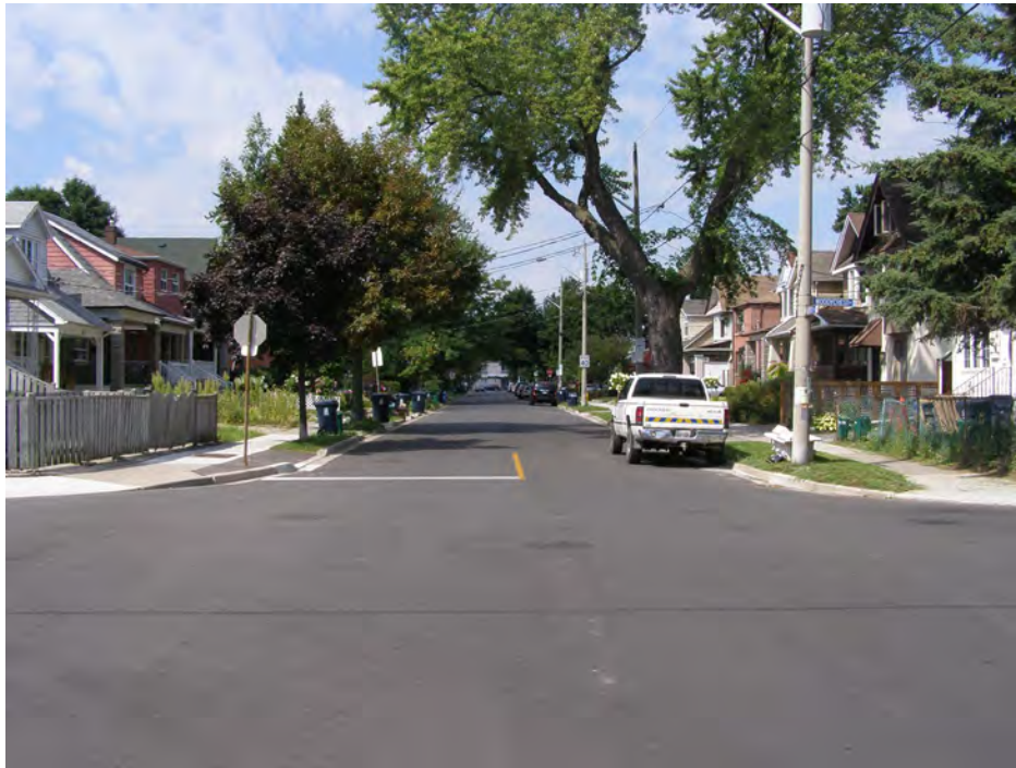
Figure 1-11 Example of a Local Road in Good Condition. Road is recently resurfaced and there are no cracks or surface distresses.
