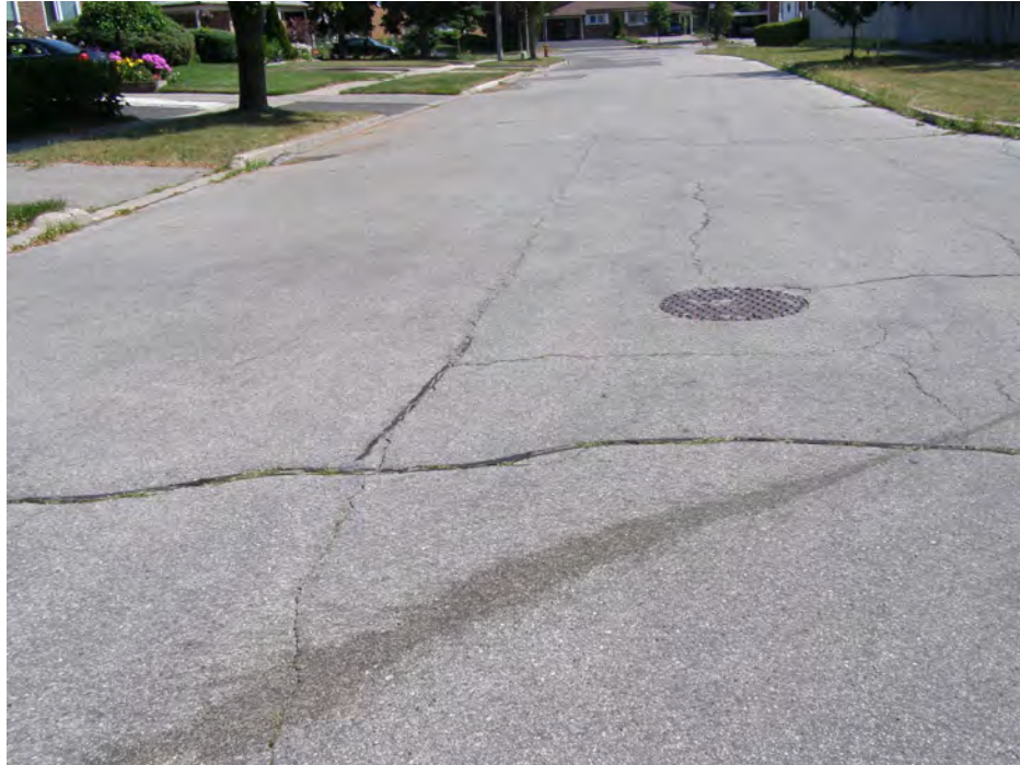
Figure 1-12 Example of a Local Road in Fair Condition. Presence of intermittent to frequent medium to large transverse and longitudinal cracks, uneven road surface.
