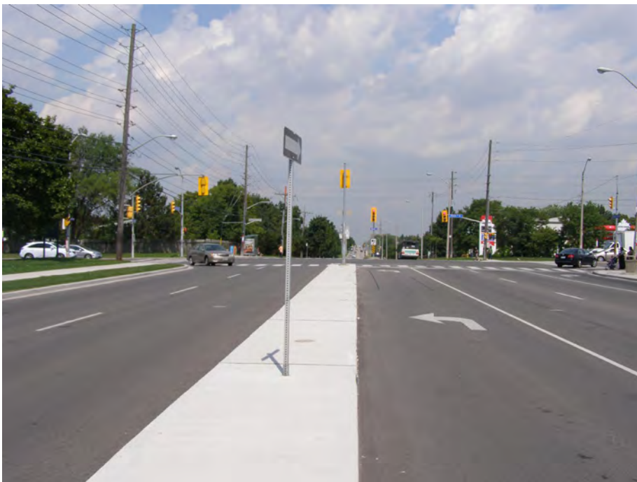
Figure 1-8 Example of an Arterial Road in Good Condition. Road is recently reconstructed and there are no cracks or surface distresses.
