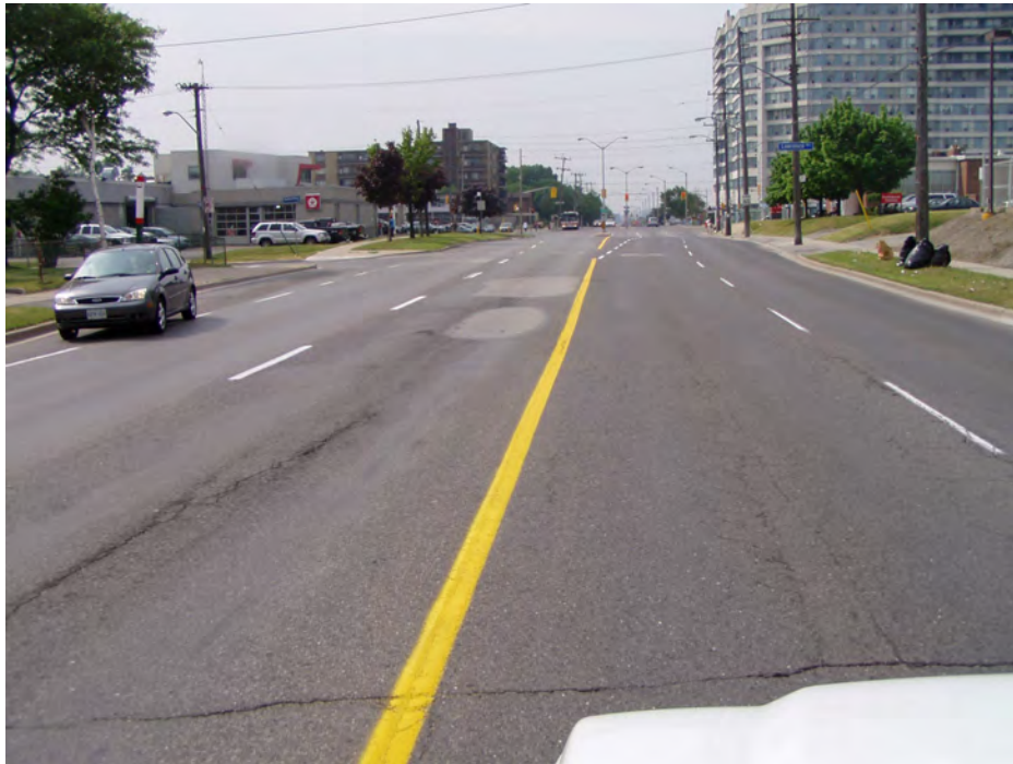
Figure 1-9 Example of an Arterial Road in Fair Condition. Presence of intermittent to frequent narrow and medium size cracks, presence of intermittent wheel path cracks and moderate rutting.
