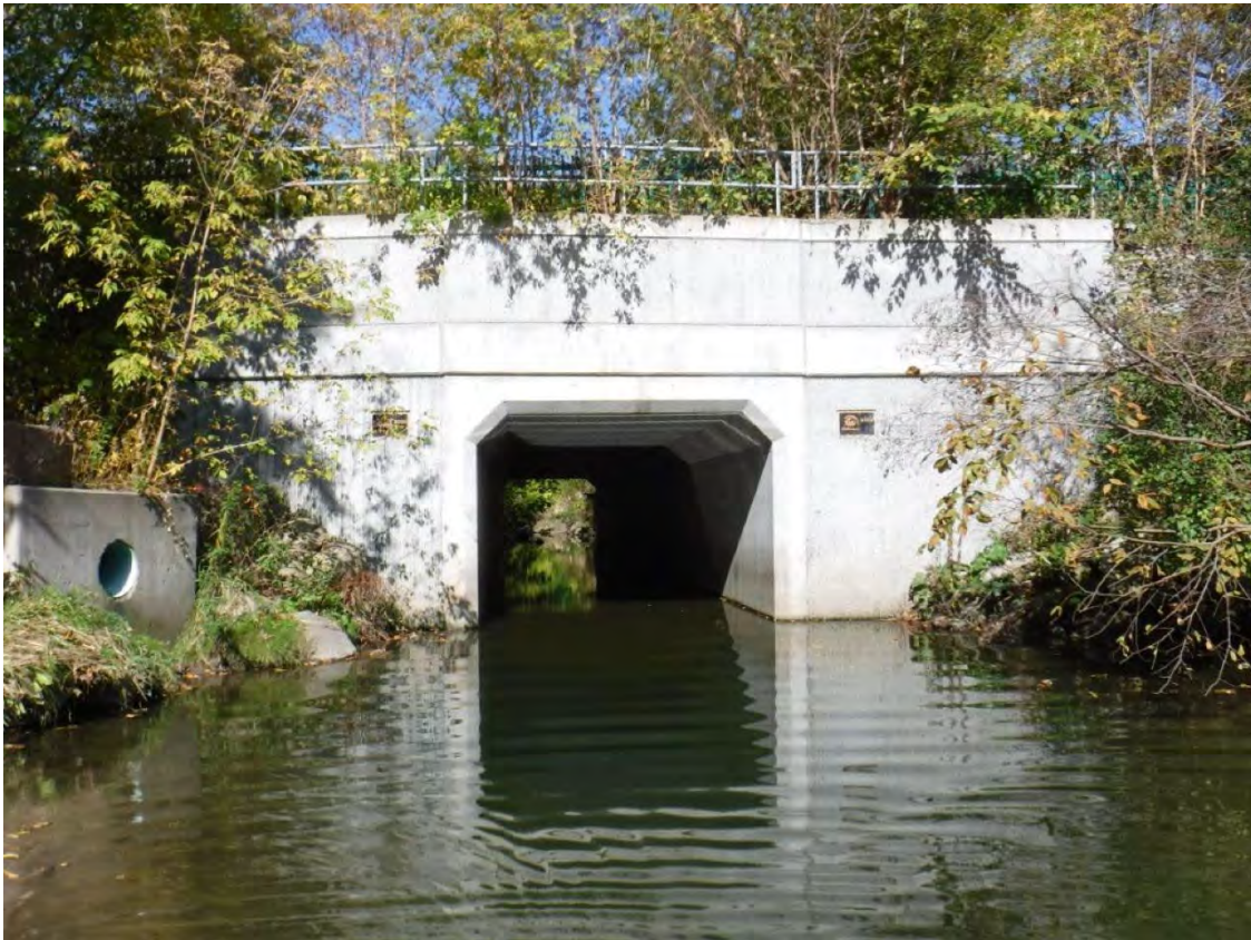
Figure 1-17 Example of a Culvert in Good Condition - ID 284 Lawrence Ave over Wilket Creek.
