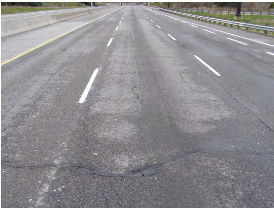
Figure 1-6 Example of Expressway in Fair Condition. Presence of intermittent to frequent narrow and medium size cracks.
