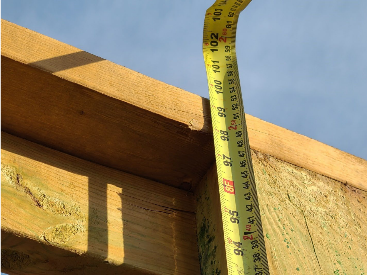
Attachment K - Front yard gate: 2.51m in height
