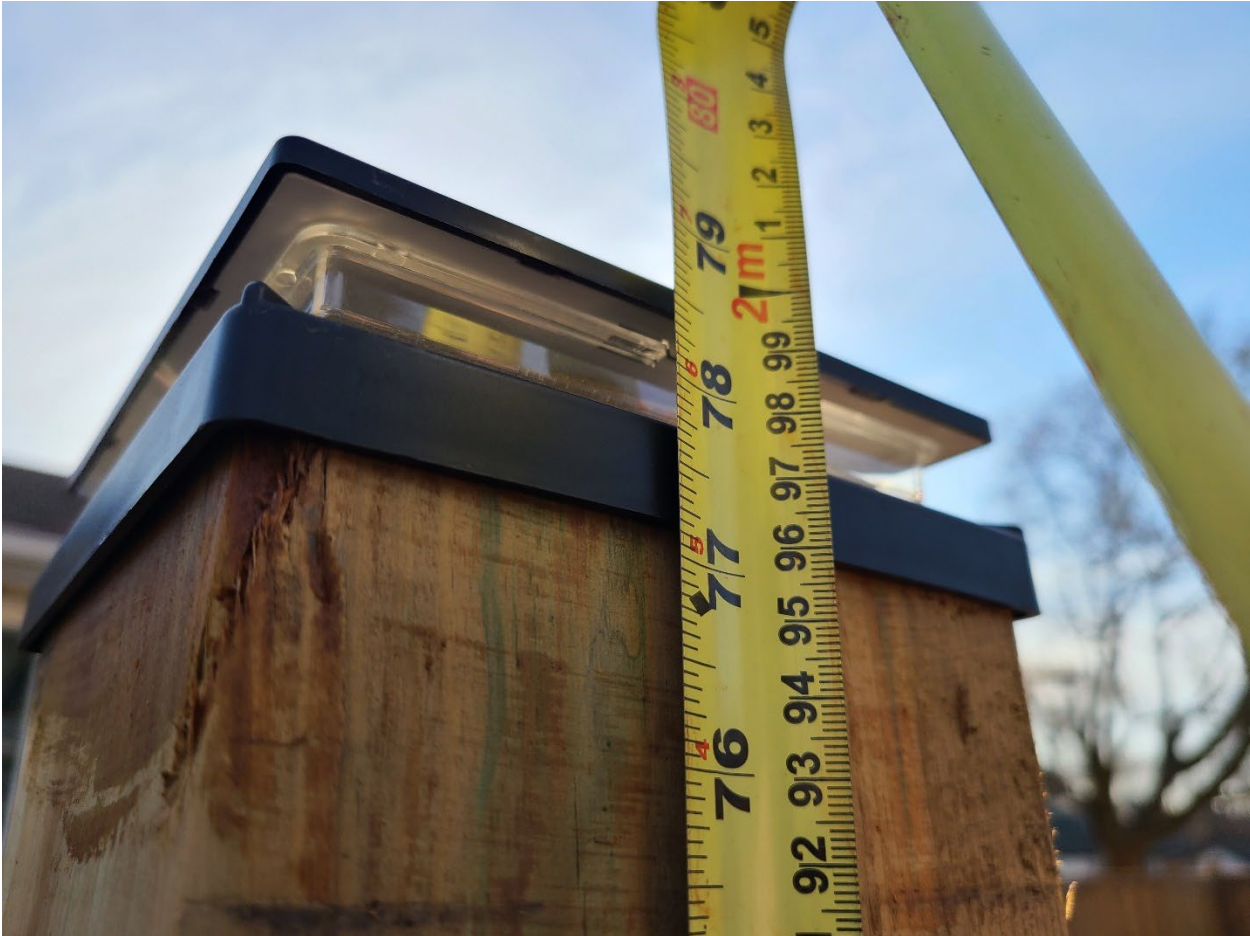
Attachment H - Side yard fence without decorative aluminum rod: 1.99m
