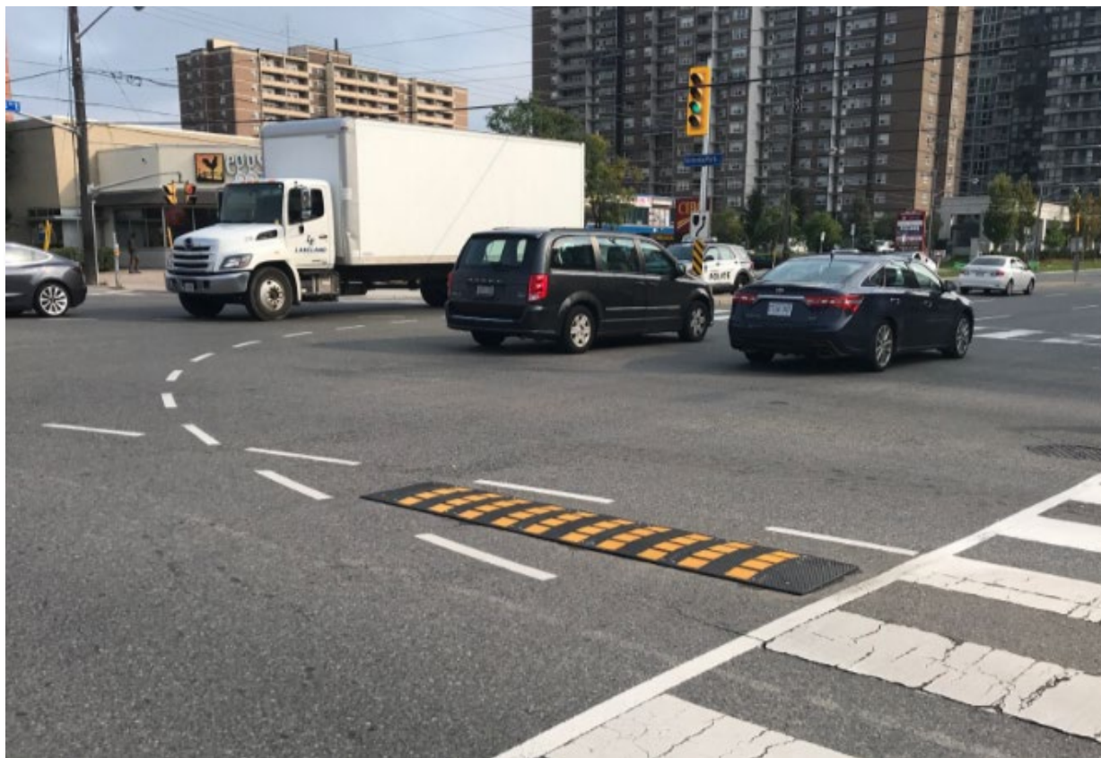
Figure 3: Curb Extension with Quick Build Materials
