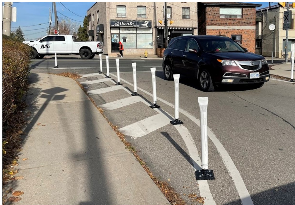
Figure 3: Curb Extension with Quick Build Materials
