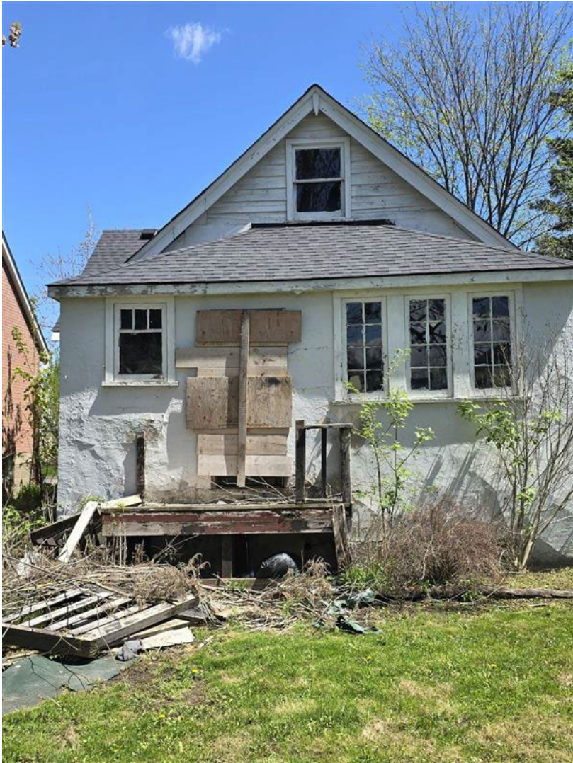
1008 Kipling Avenue Exterior
