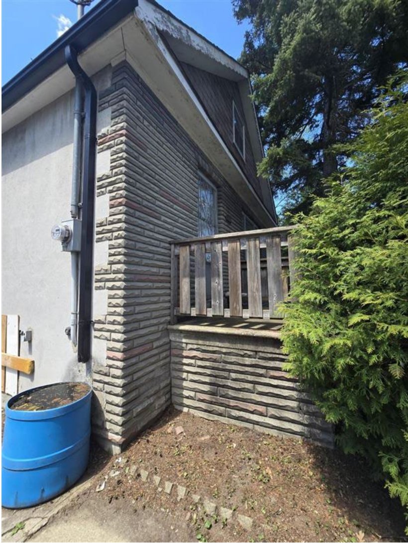
1006 Kipling Avenue Exterior
