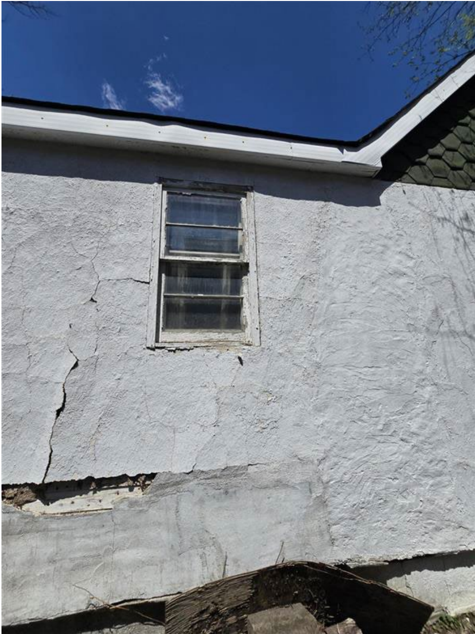
1008 Kipling Avenue Exterior
