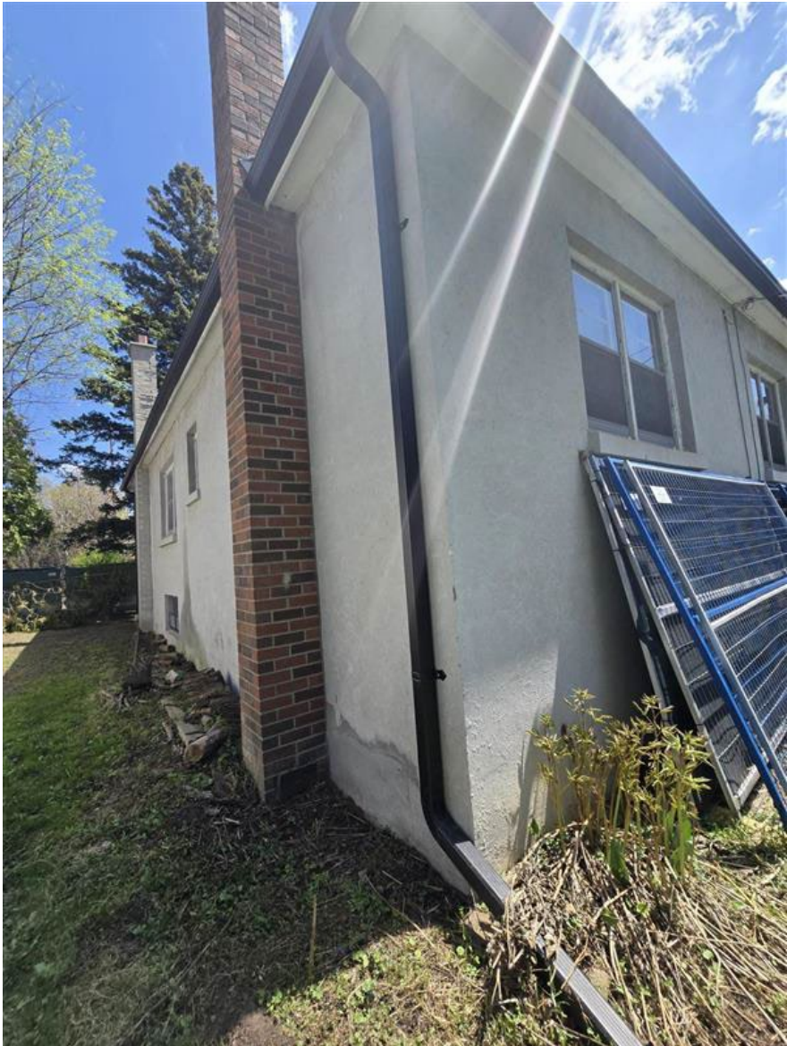
1006 Kipling Avenue Exterior
