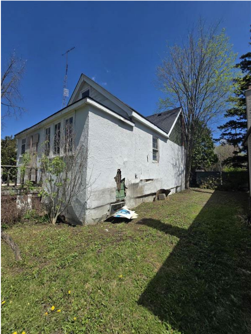
1008 Kipling Avenue Exterior
