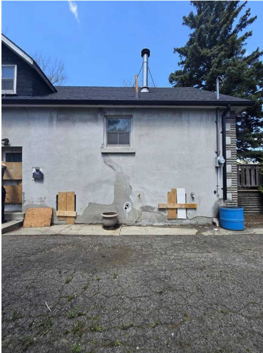
1006 Kipling Avenue Exterior
