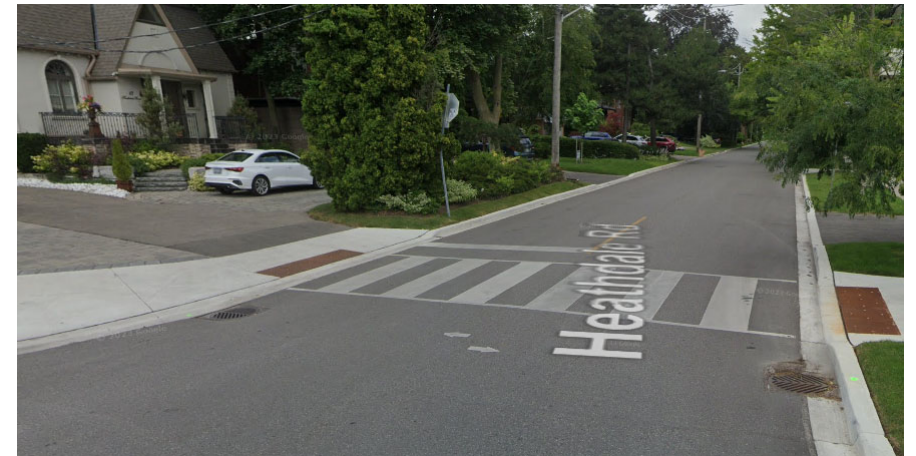
Heathdale Road and Raglan Avenue, where a portion of the driveway provides the sidewalk ramp.
