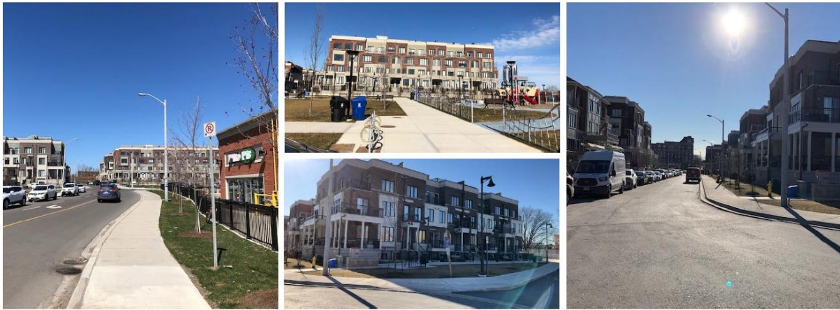
3600 3471 Lake Shore Blvd W – 4 storeys – existing context
