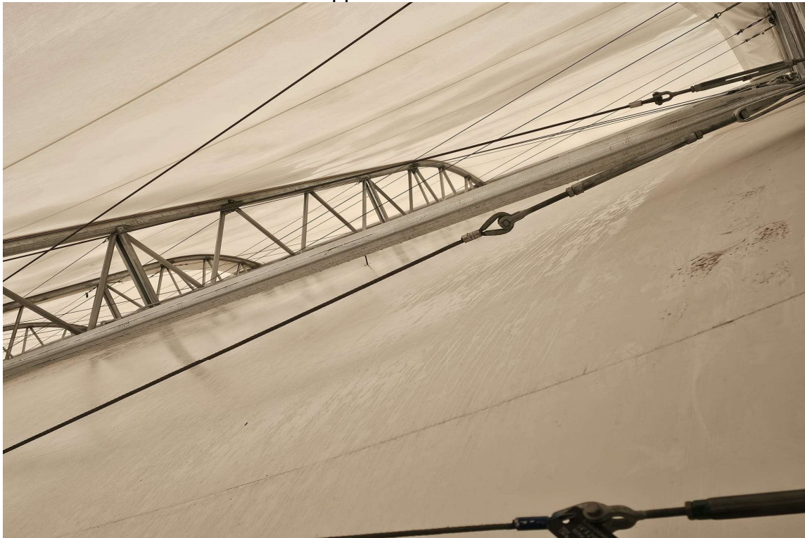
Picture 3: Additional structural supports/cables for the dome
