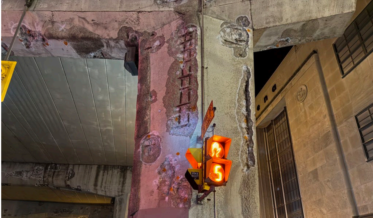
Figure 4 - Condition of reinforced concrete column at Bent 436-195
