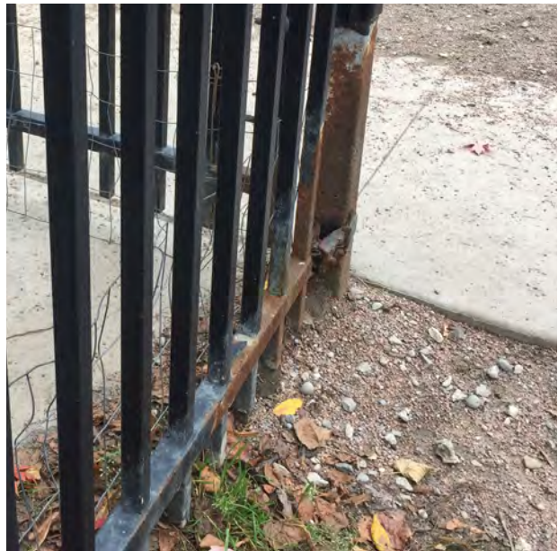
Figure 1.4. Urine Corrosion at Allan Gardens Off-Leash Area
