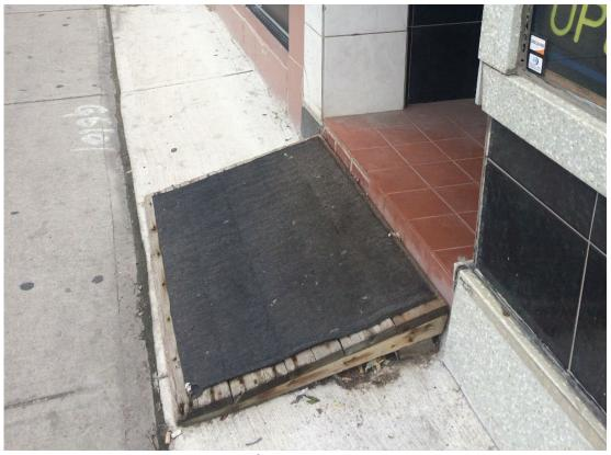
This image shows an example of improper ramp placement and design. The ramp does not align with the landing, lacks high color contrast, appears damaged, unstable, and is not slip-resistant, making it unsafe for use.
