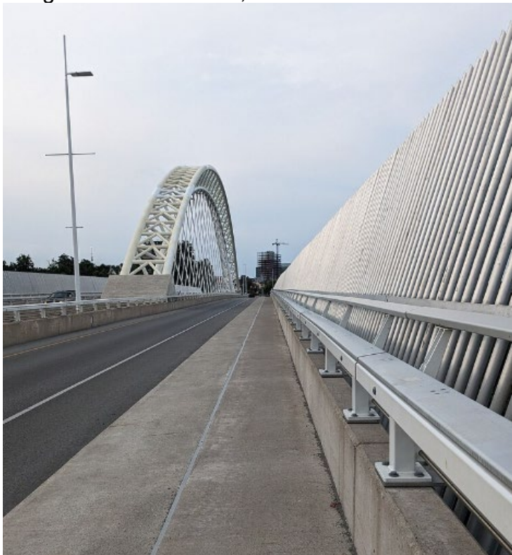
Appendix C4 – Example of Alternative 7, Angled Vertical Tubes Barrier on the Burgoyne Bridge in St. Catharines, Ontario
