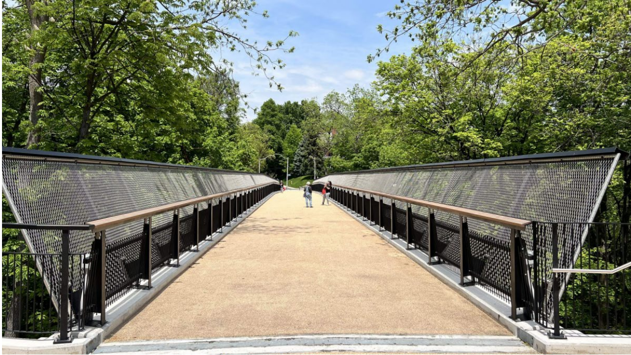
Appendix C3 – Example of Alternative 6, Angled Mesh-Link Frame on the Glen Road Pedestrian Bridge over Rosedale Valley Road (Structure ID 249)
