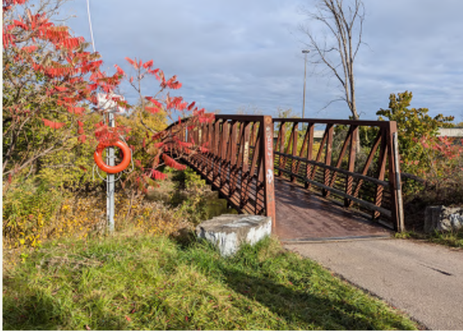
Figure 40: Bridge crossing into Crawford-Jones Park looking towards the Highway-401 underpass, connecting to the northern portion of the Humber Trail.
