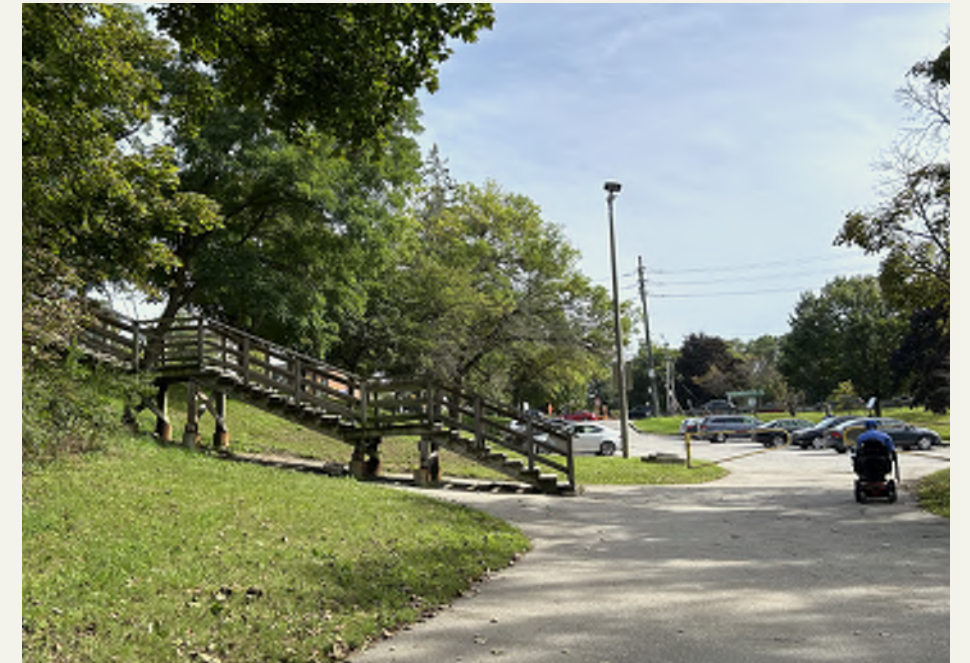
Figure 59: Cruickshank parking lot and staircase leading up to Memorial Park.
