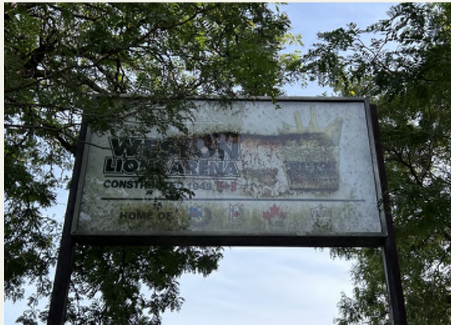
Figure 65: Dated, illegible Weston Lions Arena signage above basketball court.
