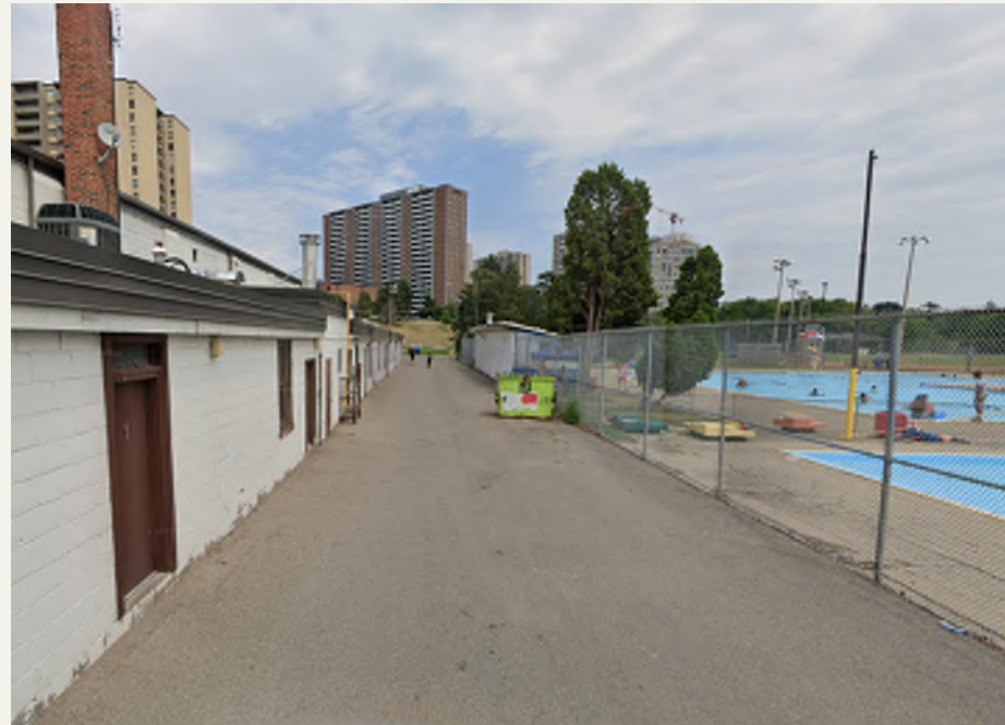
Figure 75: Alleyway between the arena and two outdoor pools.
