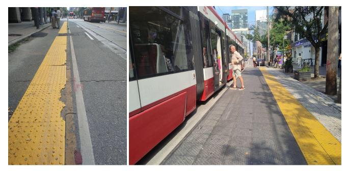
Left: Broken tactile strips at a transit stop, with part of the strip paved over a utility hole.
