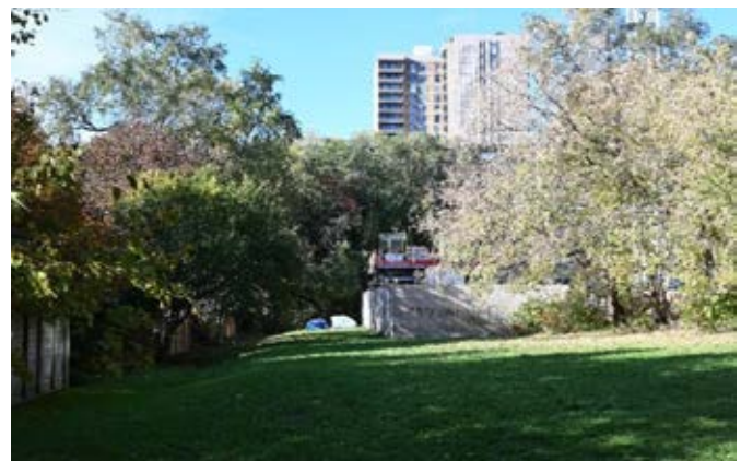
Figure 6 Culvert for stormwater management.
