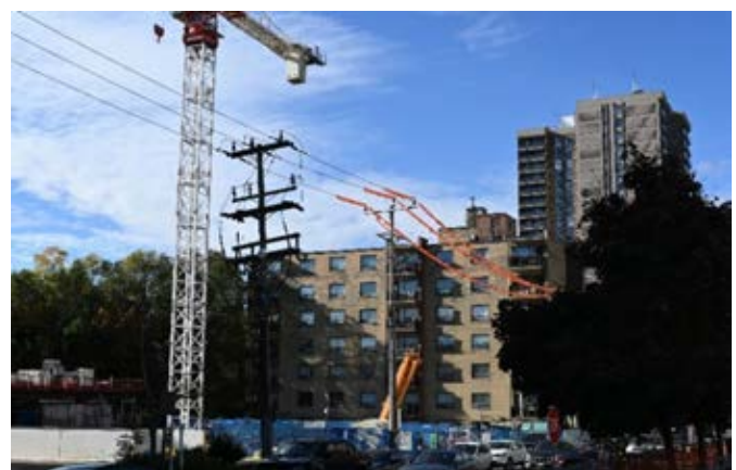
Figure 7 Utilities under construction in Marlee-Glencairn.
