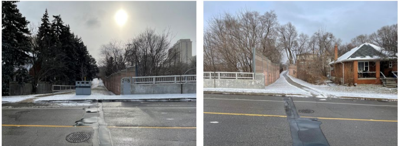
FIGURE 3-9: LACK OF PEDESTRIAN CROSSINGS ON VIEWMOUNT AVENUE - EAST SIDE OF BRIDGE
